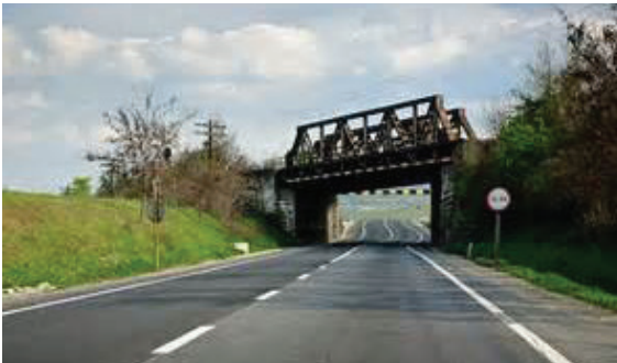
According to Cayela Wimberly from Norfolk Southern, the best highway-rail grade crossing is no crossing as shown here.
