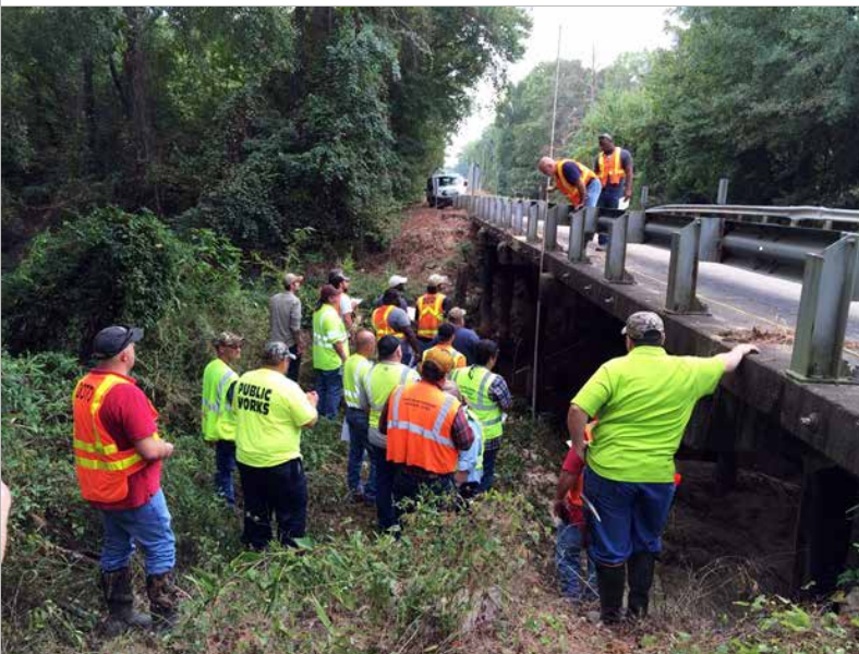
Roads Scholar #13 Inspection of Local Bridges
