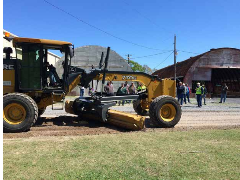
Demonstration of a motor grader operation during the Gravel Roads class at the Yambilee enter in Opelousas.
