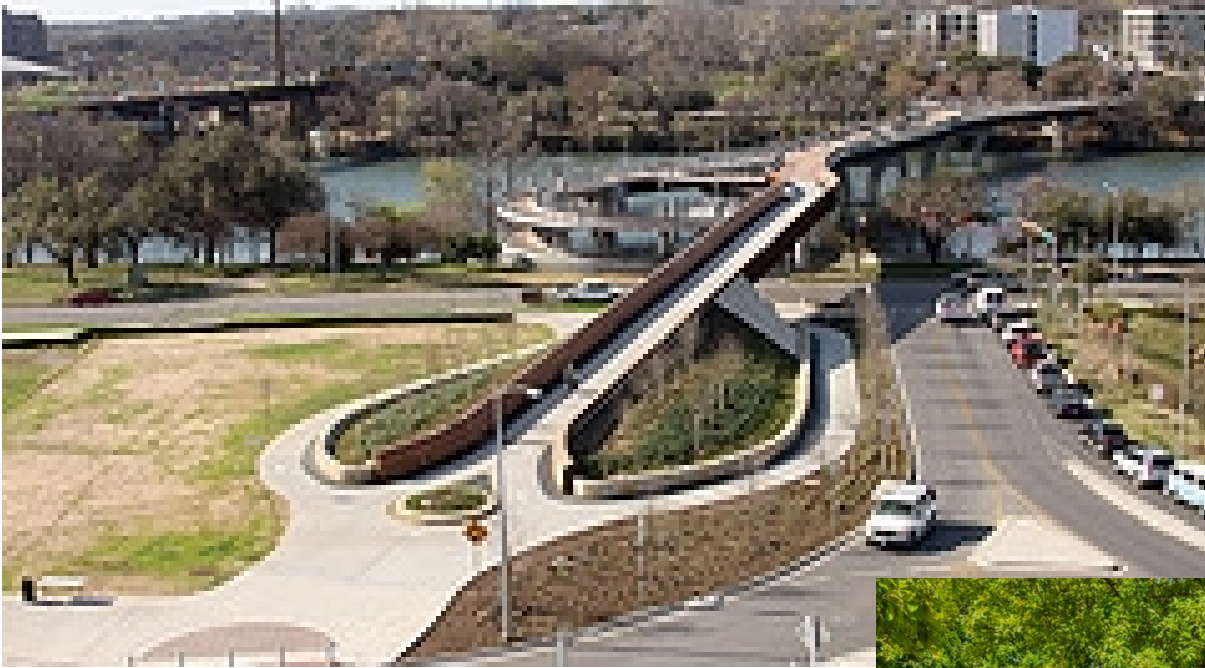
Pfluger Bicycle Bridge
