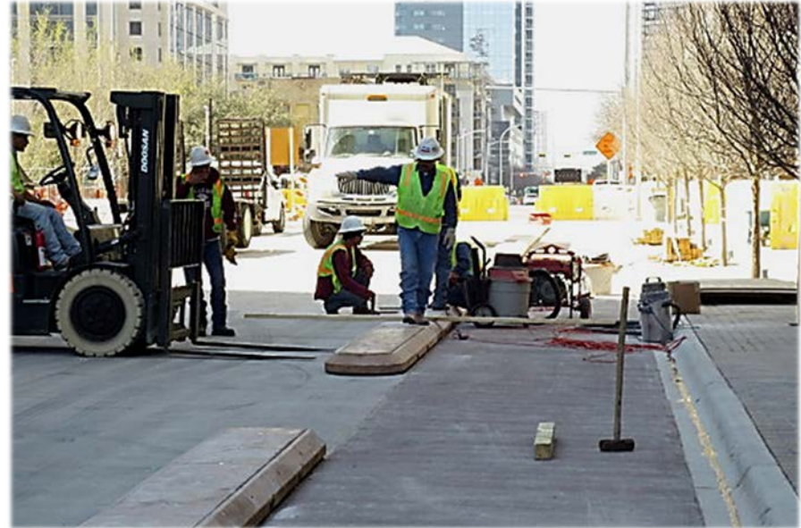
Active Transportation Program Cycle Track Project, Third Street
