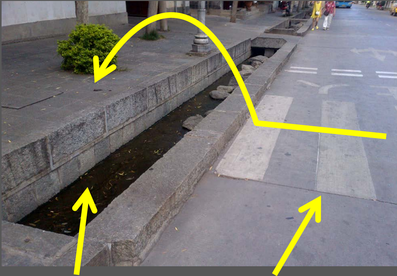
Open Drainage Ditch
