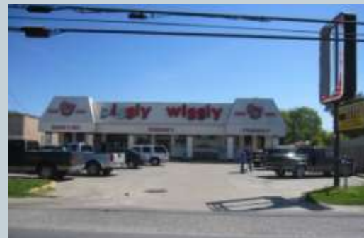
Unnecessarily wide driveways.
