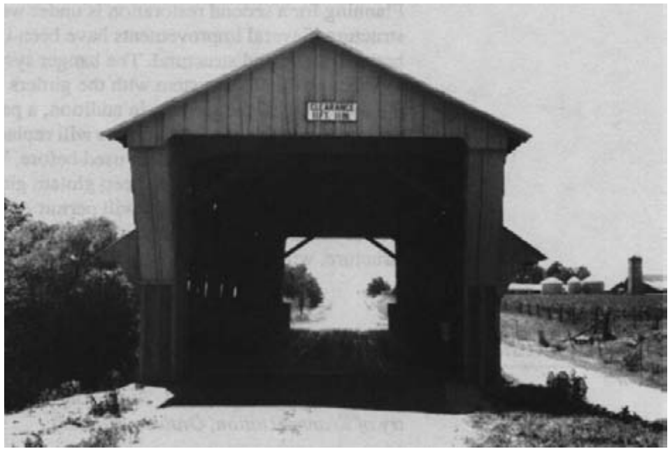
Figure 15-36. - The final result of the bridge-within-a-bridge concept. Four kneebraces to the roof system, which had been removed over the years, were reinstalled for stability and appearance. Note the improved truss alignment.
