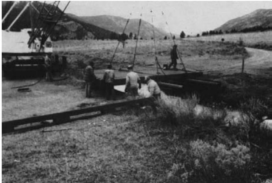
Figure 15-72. - The completed deck, resting on the well casings, is lifted into place on the abutments. Note that the curbs have been preassembled adjacent to site.
