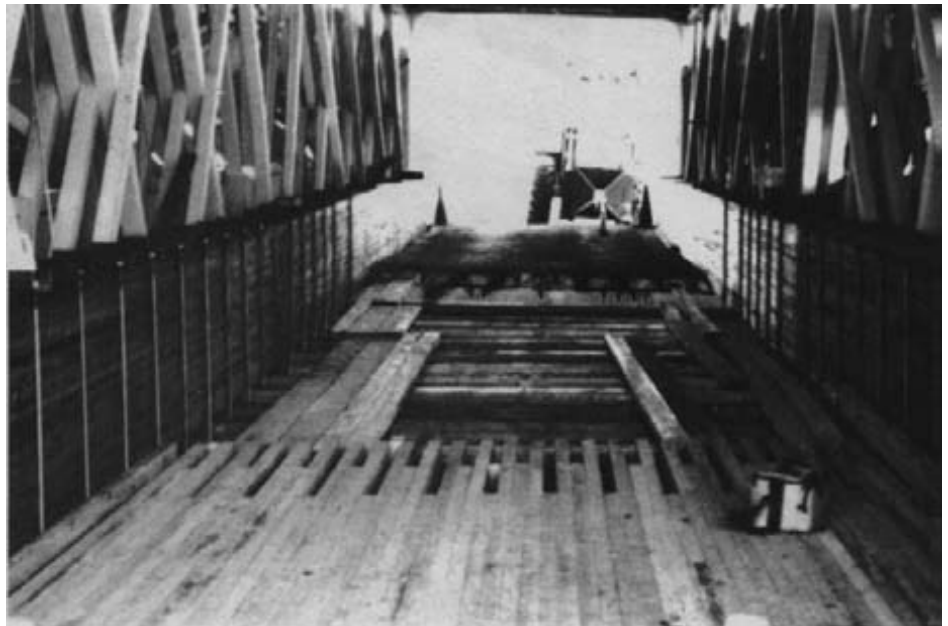
Figure 15-35. - A view inside the bridge showing the glulam girders, floorbeams, and longitudinal nail-laminated lumber floor. The existing floor, still in place at the far end of the roadway, was removed in sections to facilitate construction.
