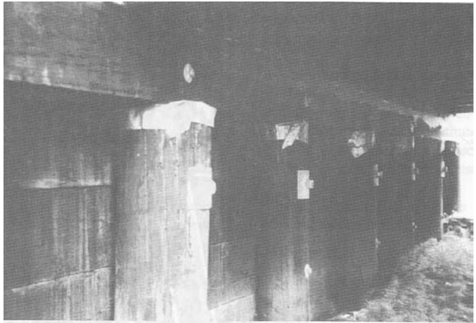
Figure 2-32.- Timber pile abutment.
