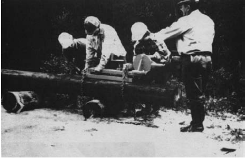
Figure 15-3. - Cutting a replacement pile section using a specially designed pile cutter.
