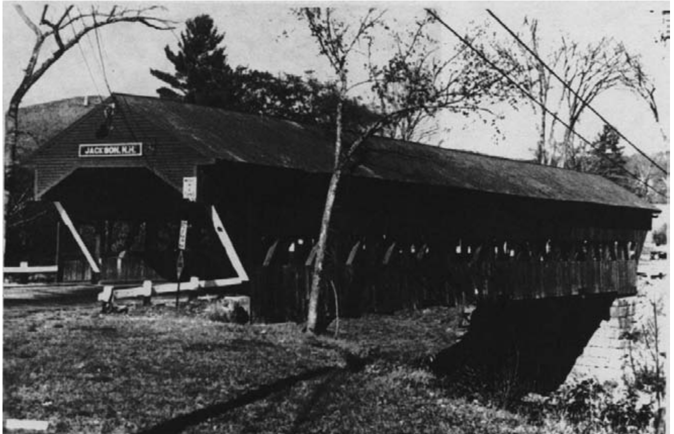
Figure 14-1. - Many covered bridges constructed of untreated timber, such as this one in New Hampshire, have lasted more than 100 years because they were protected from moisture.
