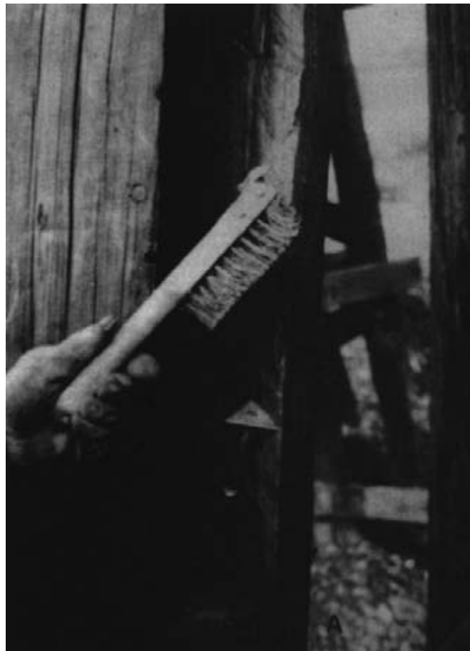
Figure 14-17. - Pile repair using pile restoration techniques. (A) The deteriorated pile area is removed as a wedge-shaped section. (photos courtesy of Osmose Wood Preserving, Inc.).
