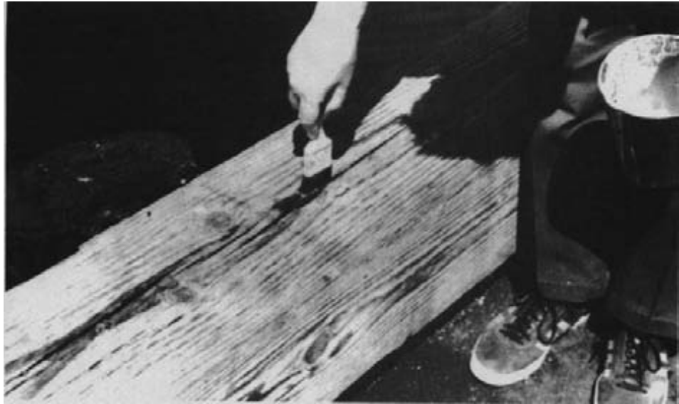
Figure 14-5. - Liquid wood preservative is applied to a check in a timber curb by brushing.
