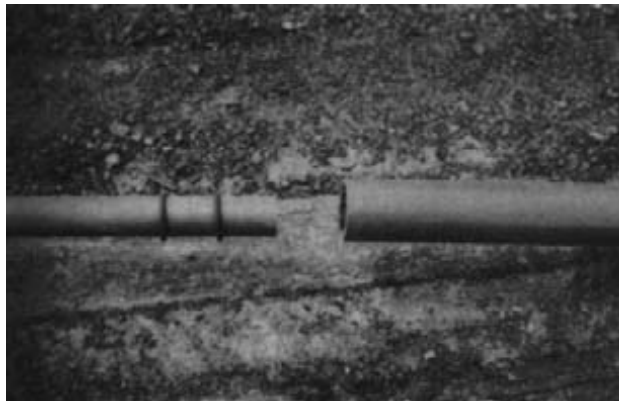
Figure 15-41. - PVC sleeve connection with neoprene O-rings.
