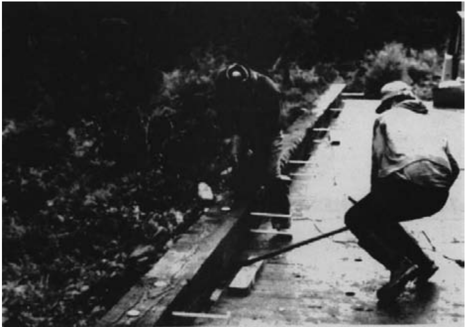
Figure 12-17. - Workers use a pry bar to align the curb for deck attachment.
