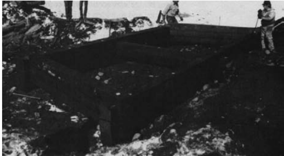
Figure 15-78.-The new crib abutment under construction using precut and creosote-treated Douglas-fir timbers. The only field fabrication involved drilling holes in the timbers for drive spikes used for connections. Such penetration of the protective envelope should have been avoided by drilling before pressure treatment (photo courtesy of Wheeler Consolidated, Inc.).
