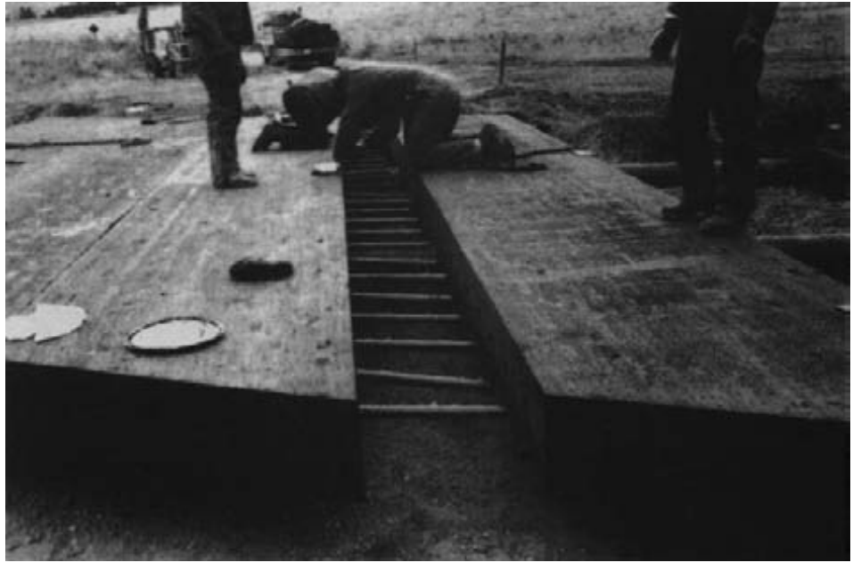
Figure 15-71. - Steel dowels are aligned before joining the fourth panel. The dowels are 1-1/2 inches in diameter, 19-1/2 inches long, and are spaced 12 inches on center.
