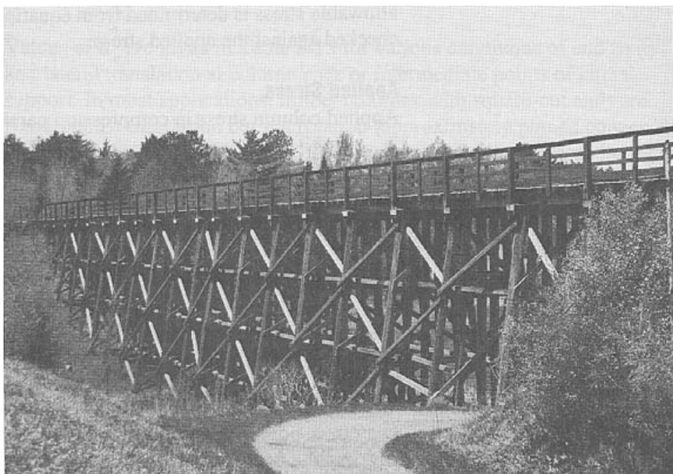
Figure 5-7.- Timber columns are common in bridge substructures such as these bents (photo courtesy Wheeler Consolidated, Inc.).
