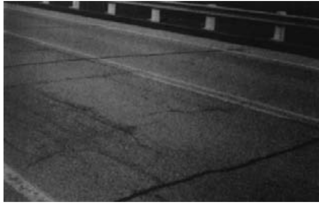
Figure 15-38. - Breakup of asphalt pavement because of delamination of the nail-laminated timber deck.
