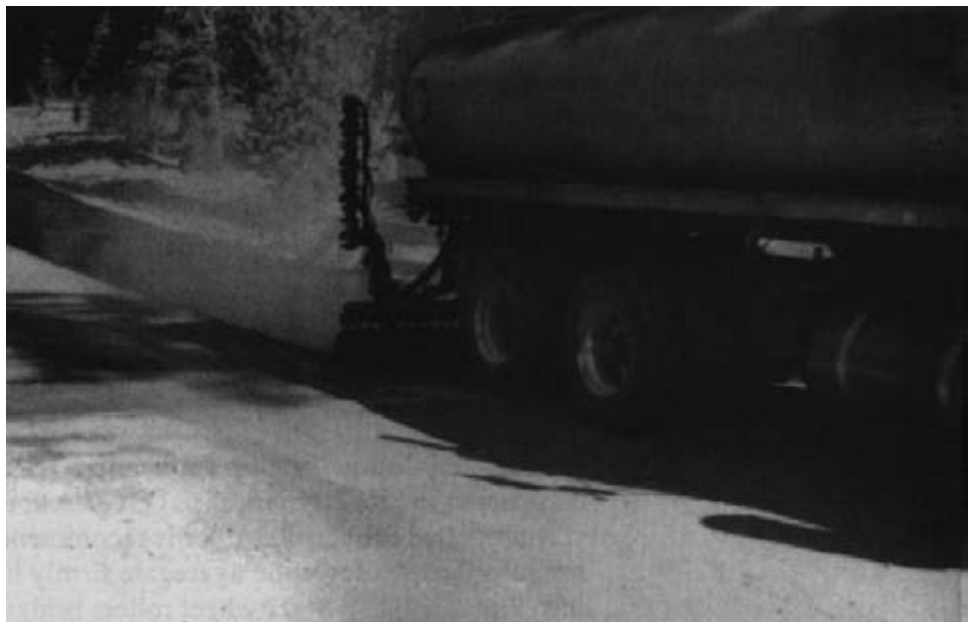
Figure 11-9. - Asphalt binder for a chip seal being applied to a timber bridge deck by an asphalt distributor truck (photo courtesy of Paul Cole, USDA Forest Service).
