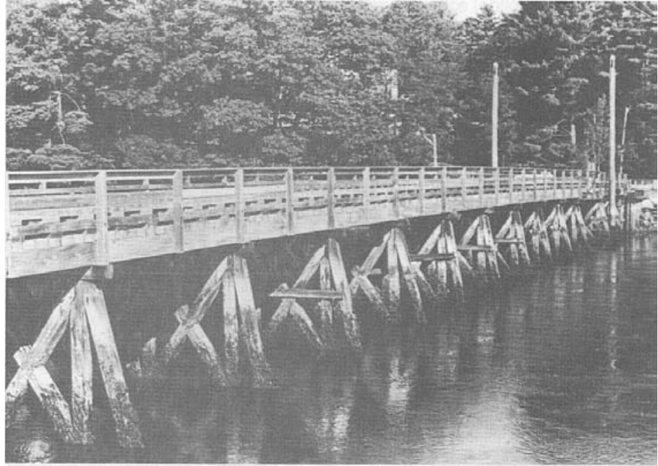
Figure 2-16.- Sewall's bridge is a timber trestle vehicle bridge in York, Maine. The bridge was built in 1933 using the same design features of the original bridge, built in 1761, that it replaced. This bridge became a designated landmark of the American Society of Civil Engineers in 1986 (photo courtesy of the American Society of Civil Engineers; Used by permission).
