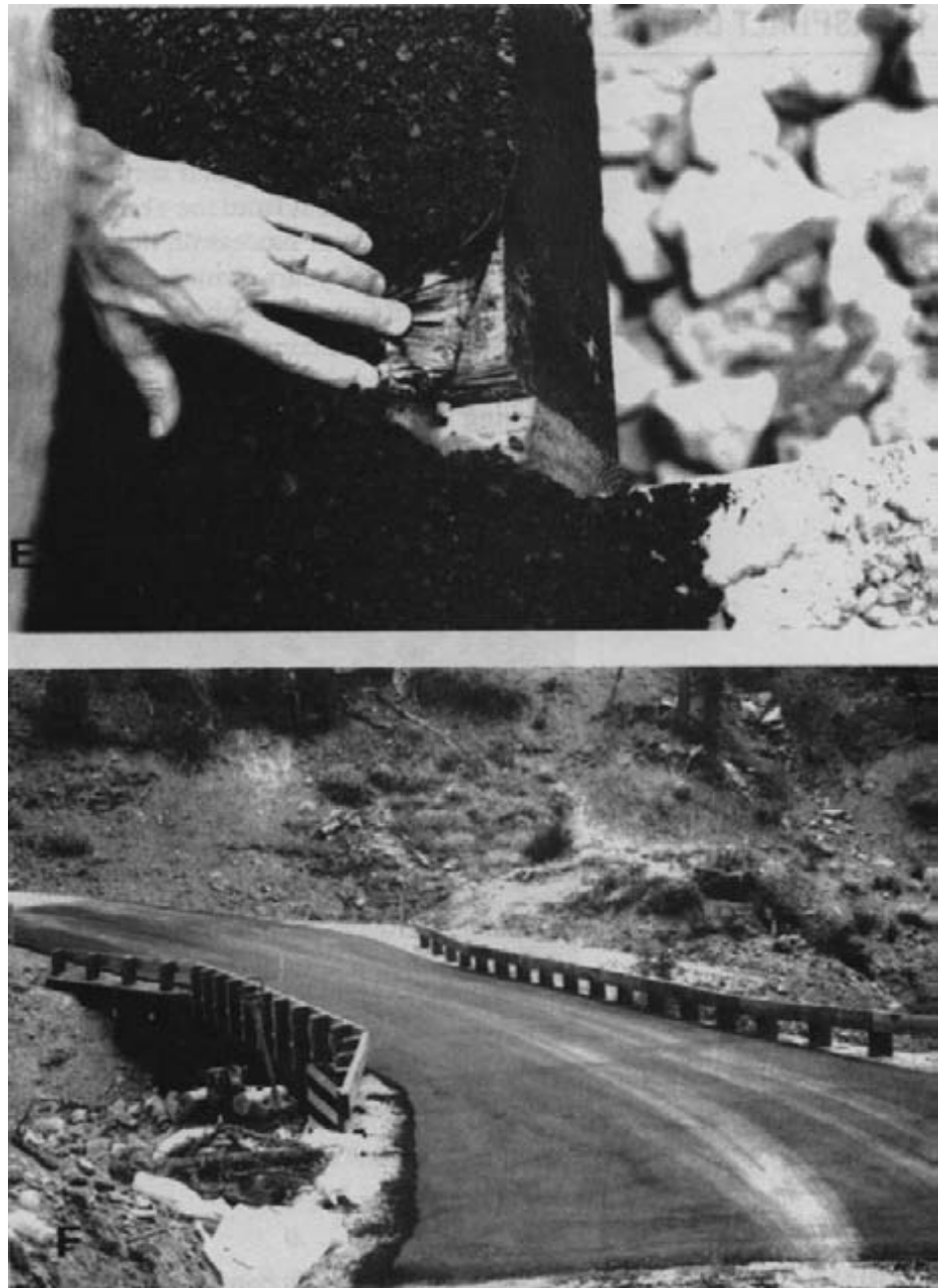
Figure 11-7. - Asphalt paving sequence on a glulam bridge deck using impregnated geotextile fabric (continued). (E) A corner of the fabric is pulled back after application of the hot asphalt, showing the bond between the rubberized asphalt on the fabric and the bridge deck. (F) The completed wearing surface (photos courtesy of Ron Vierra, USDA Forest Service).
