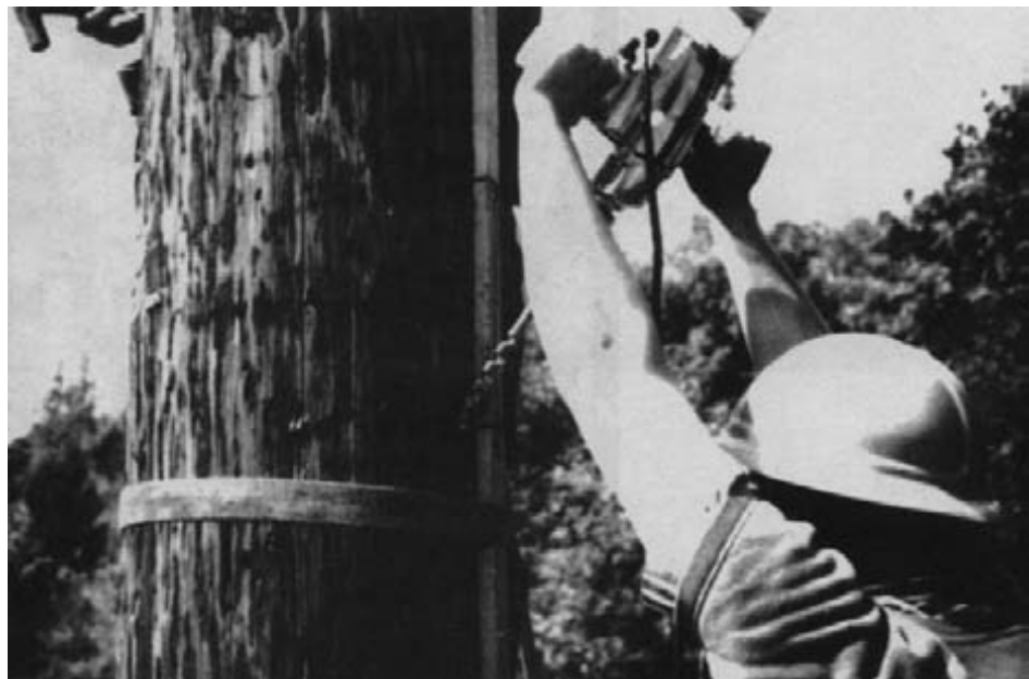
Figure 14-7. - Treating holes for fumigants in vertical members are bored at a steep downward angle (photo courtesy of Jeff Morrell, Oregon State University).
