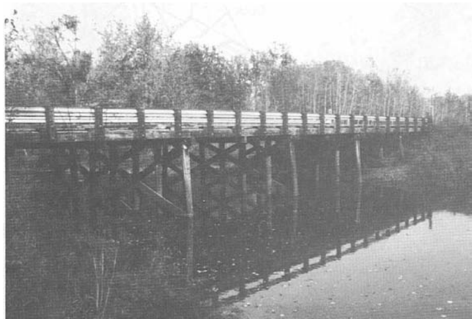
Figure 2-11.- Sawn lumber longitudinal deck bridge. Note the transverse distributor beams attached to the deck underside between bents (photo courtesy of Wheeler Consolidated, Inc.).
