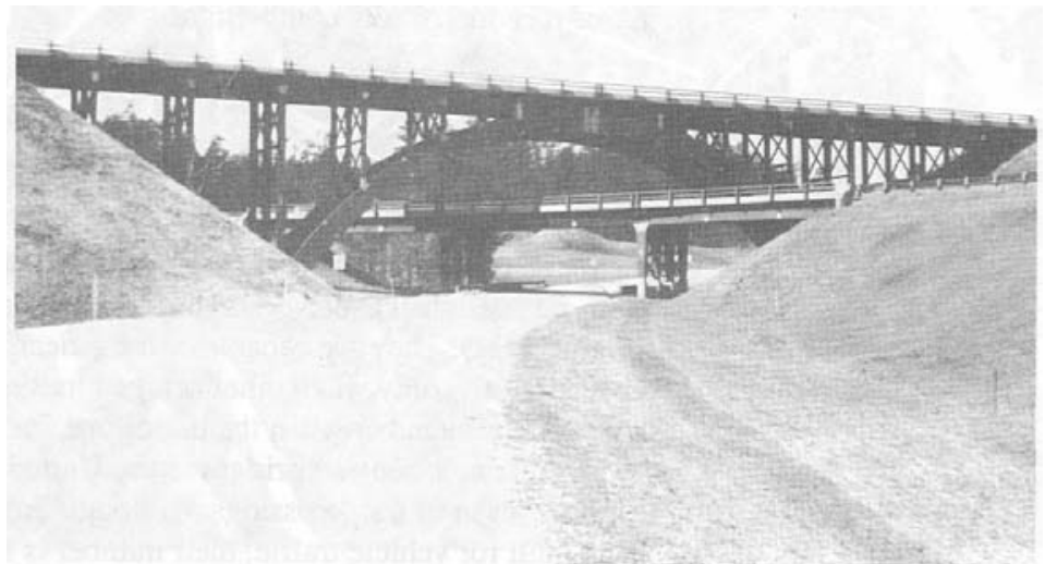
Figure 2-20.- Three-hinge glulam deck arch bridge at the Keystone Wye interchange off U.S. Highway 16, near Mount Rushmore, South Dakota. The arch spans 155 feet and supports a 26-foot-wide roadway (photo courtesy of Wheeler Consolidated, Inc.).
