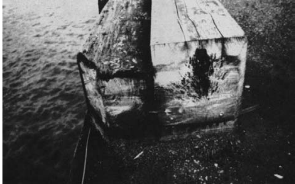
Figure 13-38. - Cross section of a timber curb, exposed by sawing, reveals interior decay resulting from seasoning checks in the upper surface.
