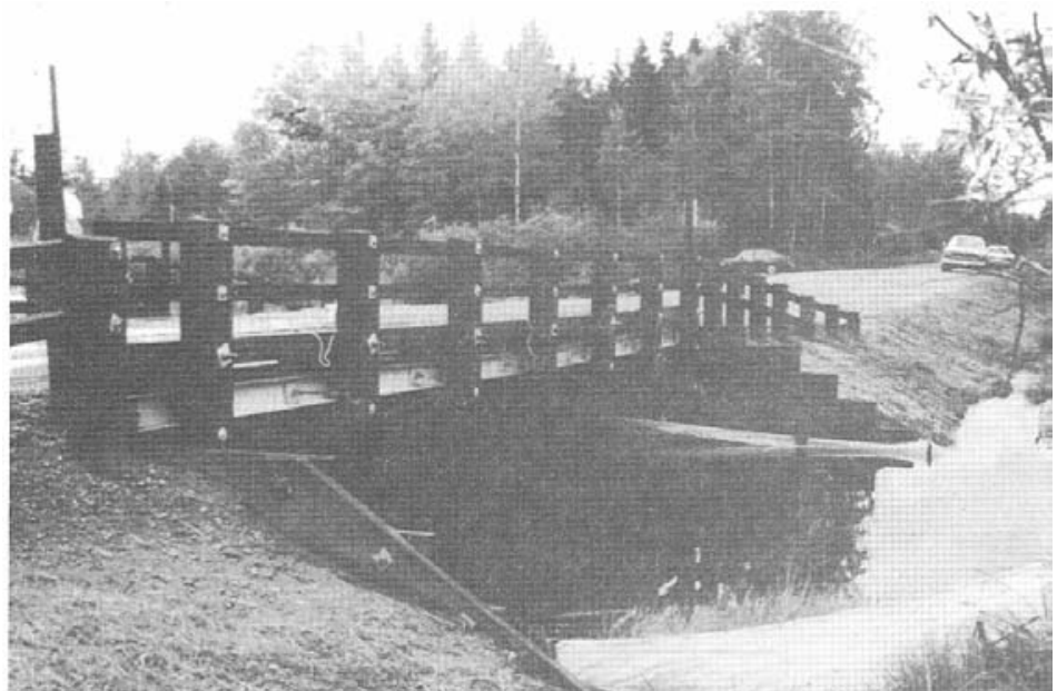
Figure 9-2. - Stress-laminated deck bridge built over Iron River on the Chequamegon National Forest in 1988.
