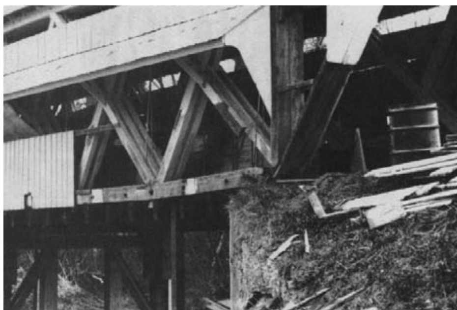
Figure 15-33. - Broken lower chords at two of the four corners prompted the replacement of some existing truss members.
