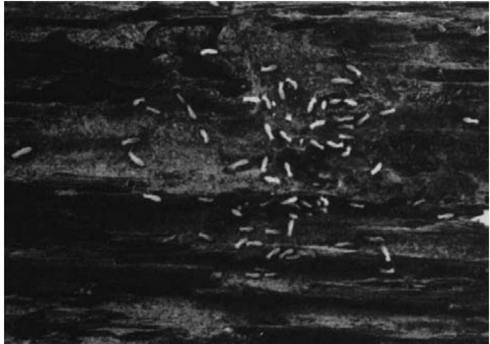
Figure 13-9. - Subterranean termites and the wood damage they cause. Note the frass and debris accumulations in the tunnels (photo courtesy of USDA Forest Service, Forest Sciences Laboratory, Gulfport, Mississippi).
