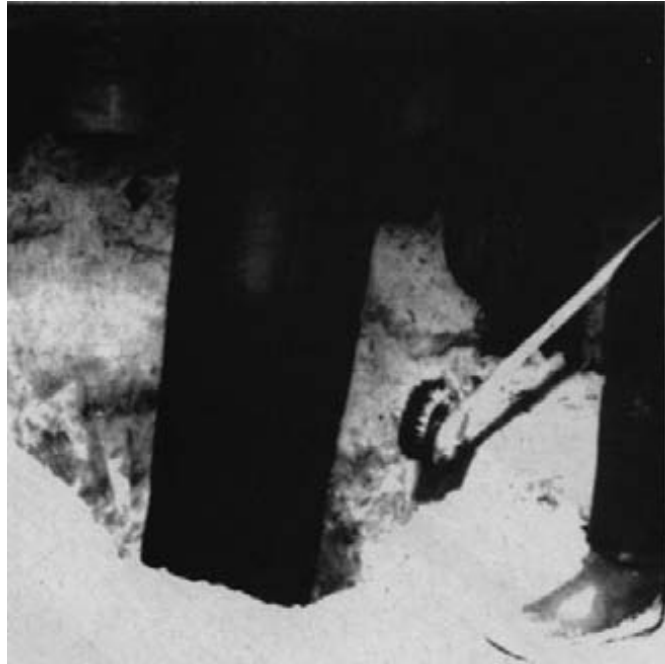
Figure 14-6. - Paste wood preservative is applied to a timber pile around the groundline. Note the wrapping material at the upper end of the treated section (photo courtesy of Osmose Wood Preserving, Inc.).
