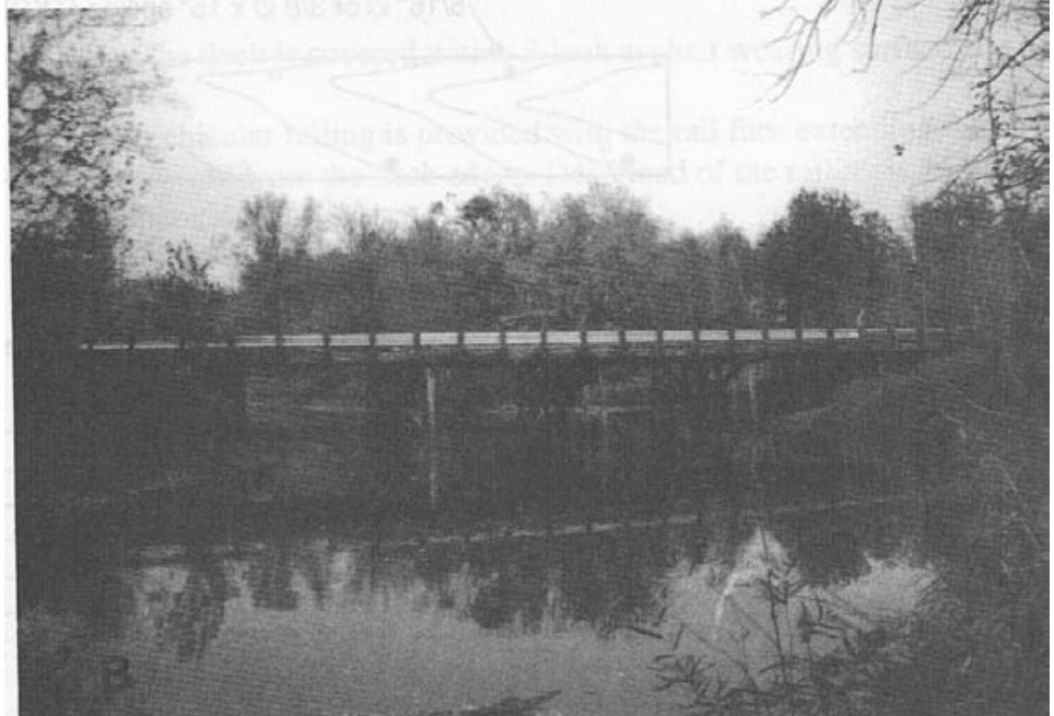
Figure 8-12. - Panelized longitudinal nail-laminated deck bridges (continued). (B) Typical multiple-span bridge configuration (photos courtesy of Wheeler Consolidated, Inc.).
