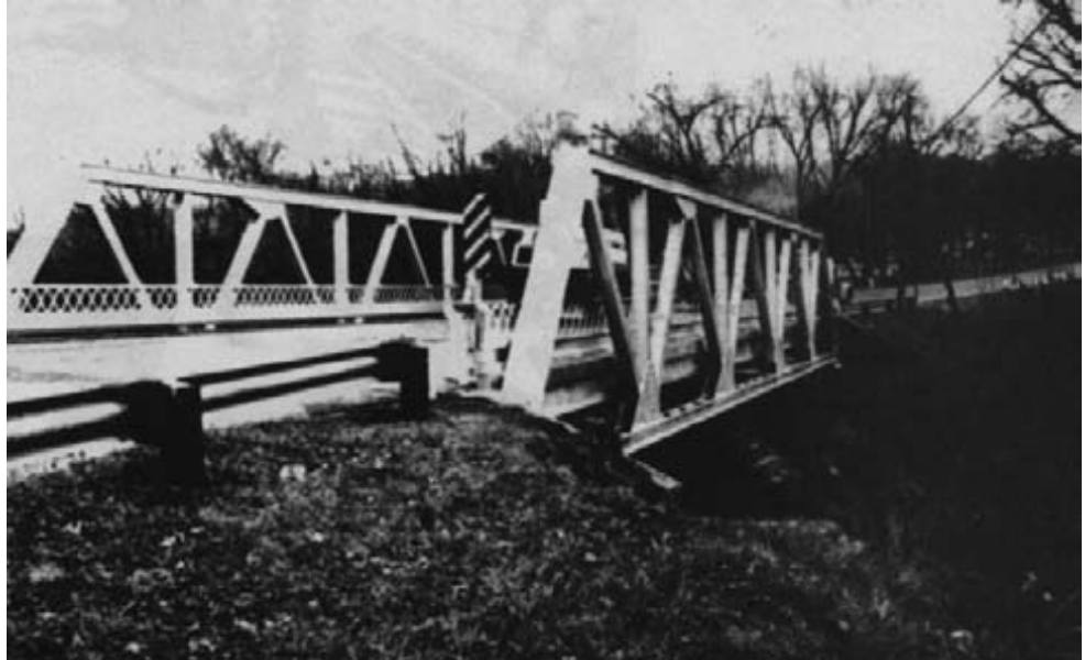
Figure 15-47. - The existing bridge was a steel truss, 96 feet long, with a 26-foot roadway width. The noncomposite concrete deck was supported by steel stringers (WF16 x 50) spaced 4 feet 6 inches on center. The stringers were supported by steel floor beams (WF30 x 116).
