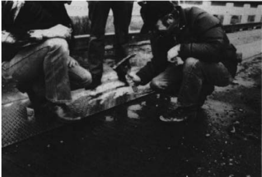
Figure 13-34.- After treating an inspection hole in a bridge deck with liquid wood preservative it is plugged with a treated wood dowel (photo courtesy of Frank Muchmore, USDA Forest Service).
