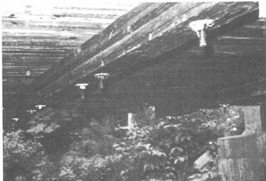
Figure 8-4. - Transverse glulam stiffener beam attached to the underside of a longitudinal glulam deck bridge (photo courtesy of Dave Nordenson, USDA Forest Service).
