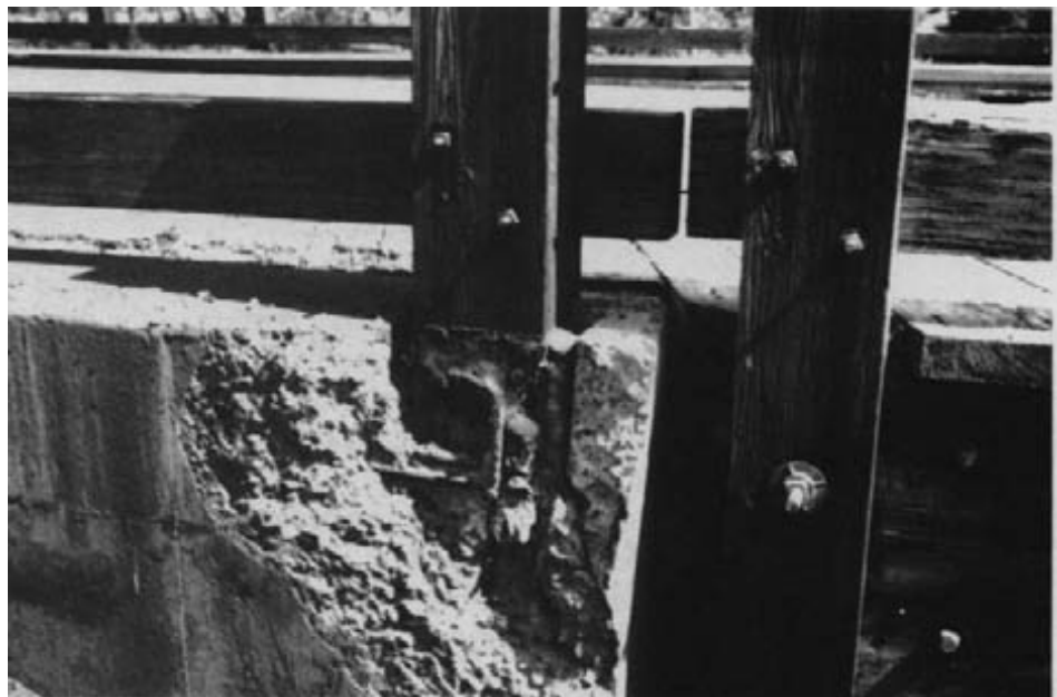
Figure 13-48. - Decay in a timber railpost embedded in concrete at the abutment. Concrete spalling was caused when water trapped in the post cavity was subjected to freeze-thaw cycles.
