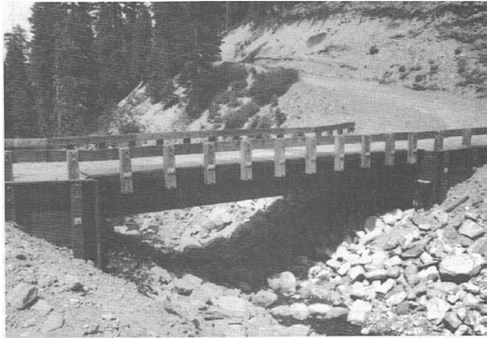
Figure 6-12. - A timber bridge with sharply curved approach roadways. Trucks crossing the bridge can produce centrifugal forces that affect the bridge superstructure and substructure.
