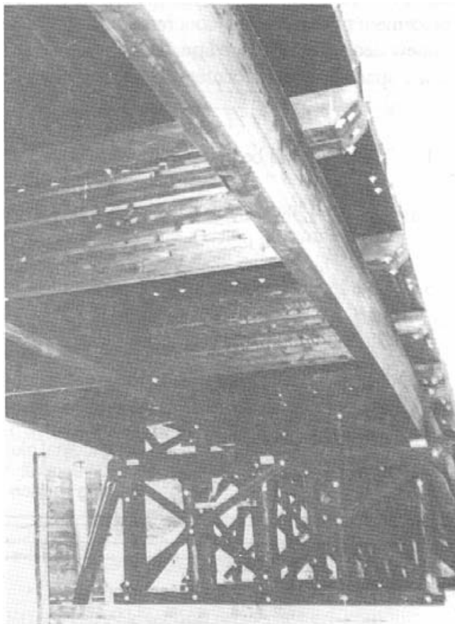
Figure 8-19. - Longitudinal glulam deck on transverse glulam floorbeams.
