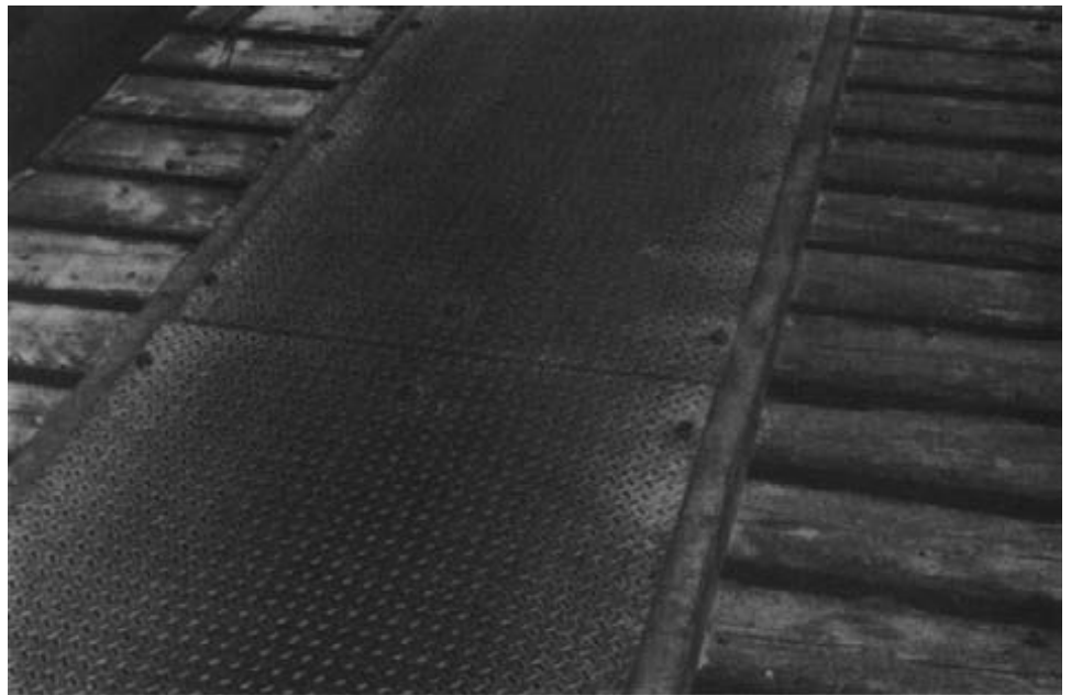
Figure 11-21. - Typical checkered surface pattern on steel running plates.
