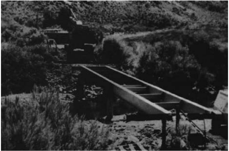
Figure 15-62. - A portion of the final paint coat has been applied to the steel and the new treated-timber abutments are in-place. The backhoe is positioned to lift the longitudinal glulam panels for the far side approach span.
