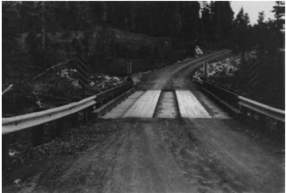
Figure 11-25. - Timber bridge deck with lumber running planks.
