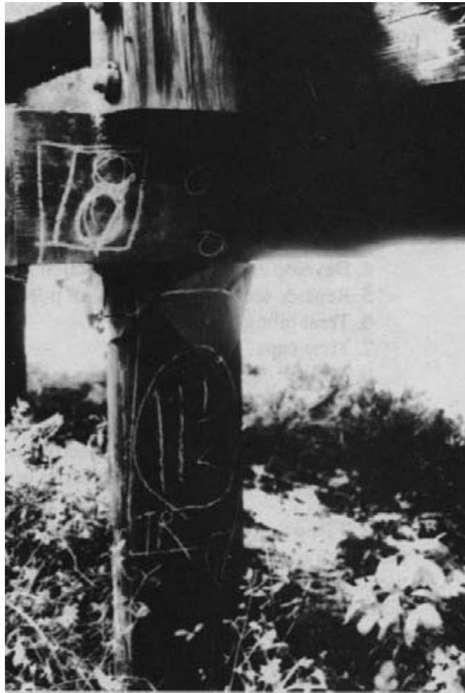
Figure 15-1. - Typical investigative borehole pattern.
