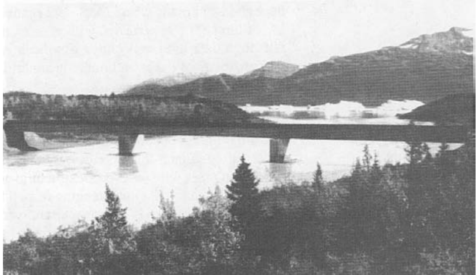
Figure 2-7.- Glulam beam bridge over Dangerous River, near Yukatat, Alaska. This bridge consists of three 143-foot spans, each of which is supported by four glulam beams that are 91-1/2 inches deep (photo courtesy of the Alaska Department of Transportation and Public Facilities).
