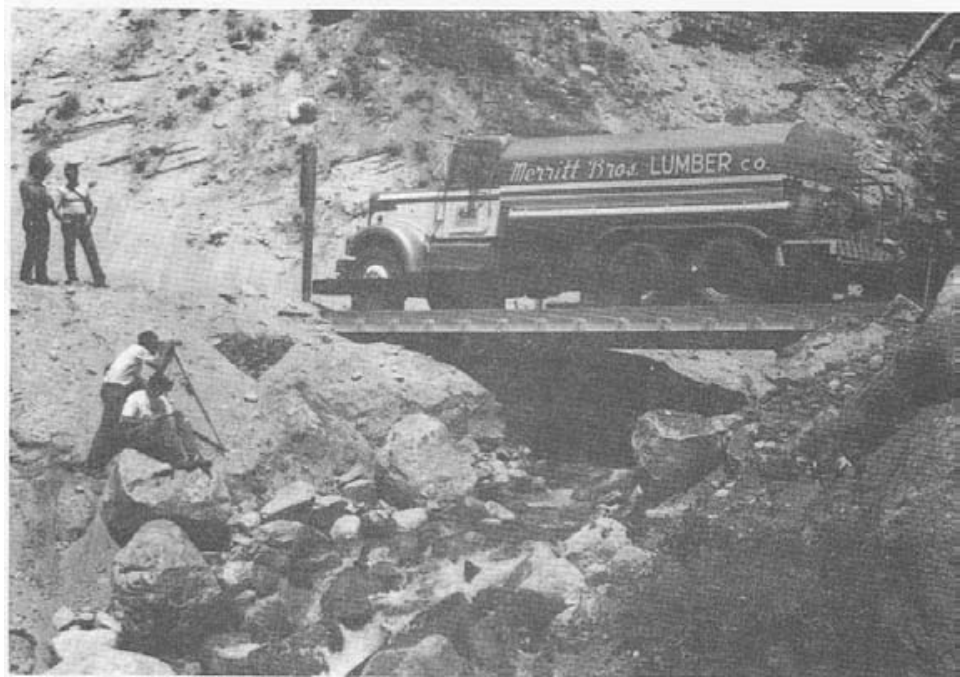
Figure 9-5. - Load test of the Zuni Creek stress-laminated deck on the Idaho Panhandle National Forests.
