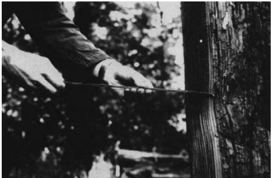
Figure 13-31. - Use of a shell depth indicator, illustrated with a portion of the member removed. The tool is inserted into an inspection hole and moved along the hole sides to feel for decay voids.
