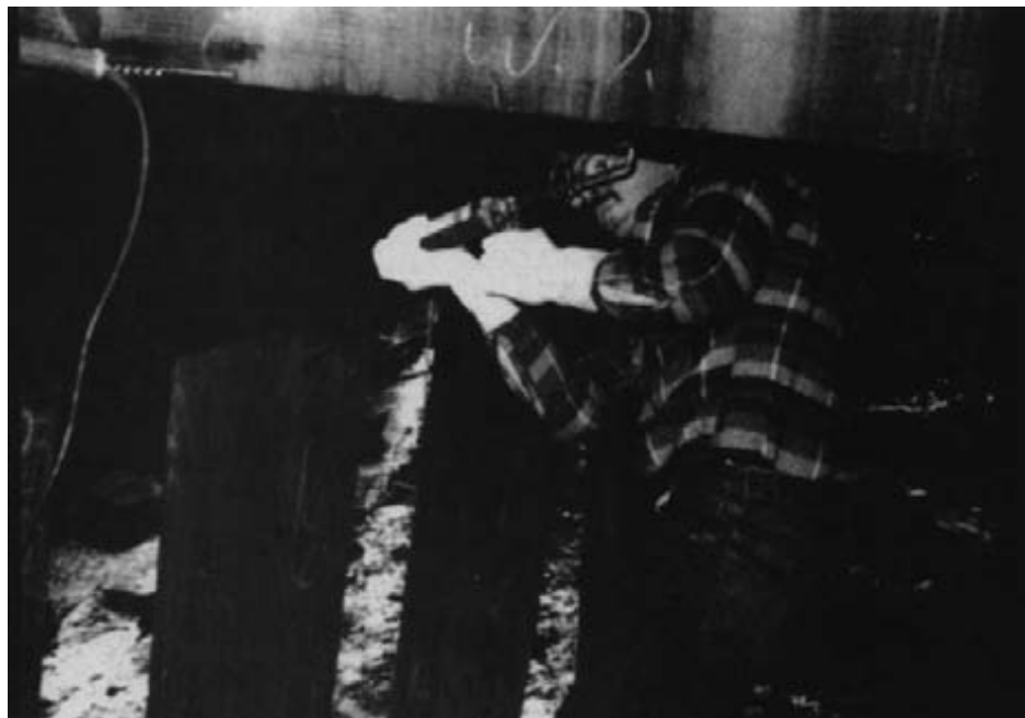
Figure 14-19. - Epoxy is manually injected between a timber pile and cap using a caulking gun (photo courtesy of Osmose Wood Preserving, Inc.).
