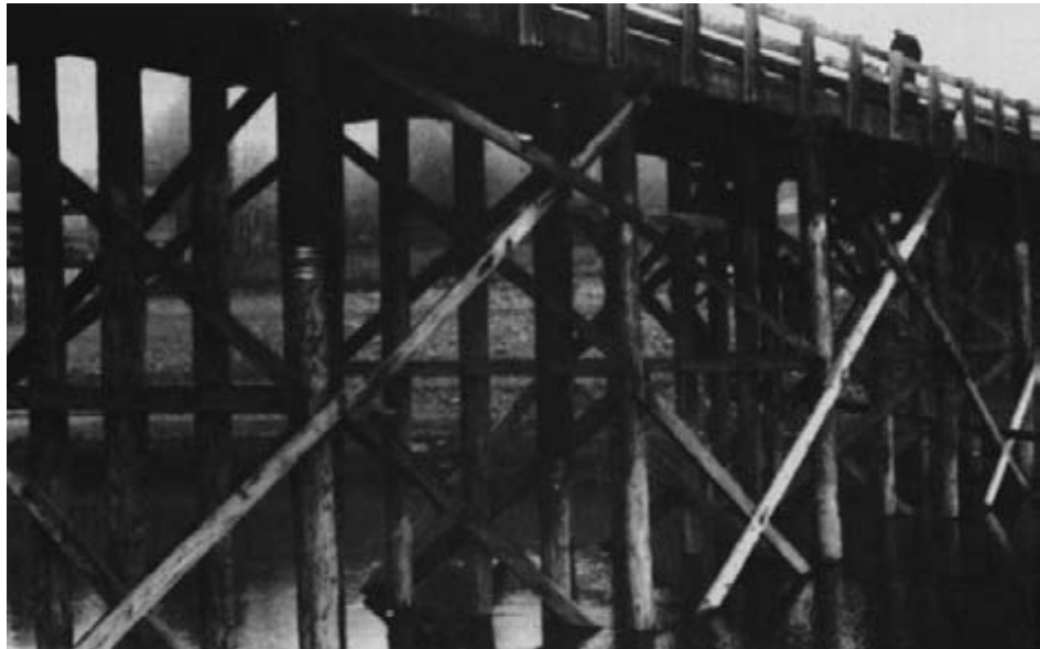
Figure 15-17. - Pile bents after replacement of deteriorated sections by pile posting.
