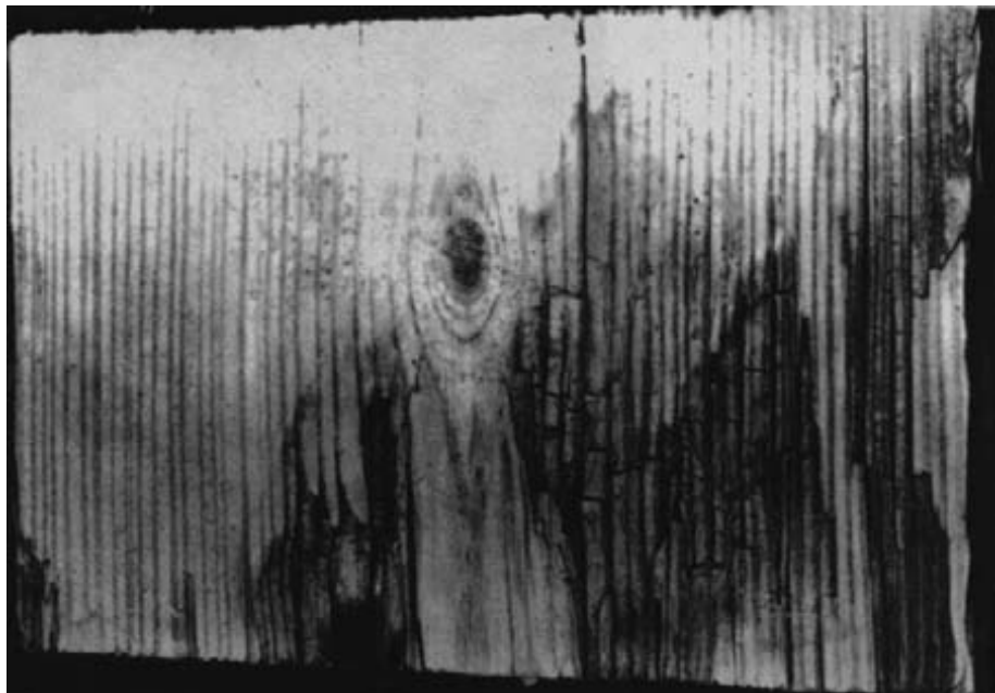
Figure 13-4. - Wood infected with brown rot fungi in an advanced stage. The decayed wood has a darkened color with a cracked, brittle surface that resembles charred wood.
