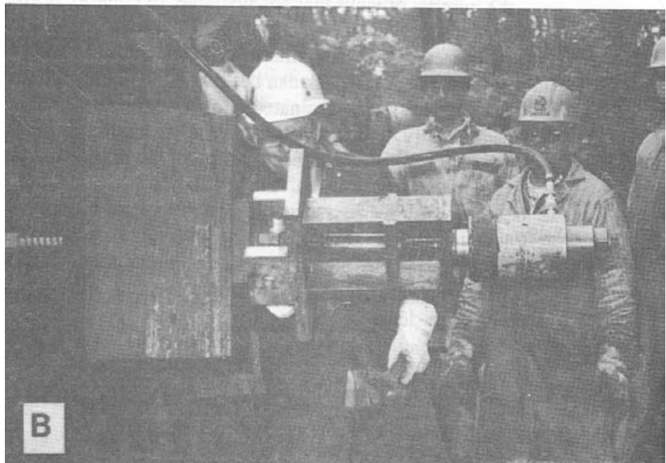
Figure 9-14. - Types of hollow core jacks used for stress-laminated bridges. (A) With a built-in ratchet. (B) With a steel chair assembly.
