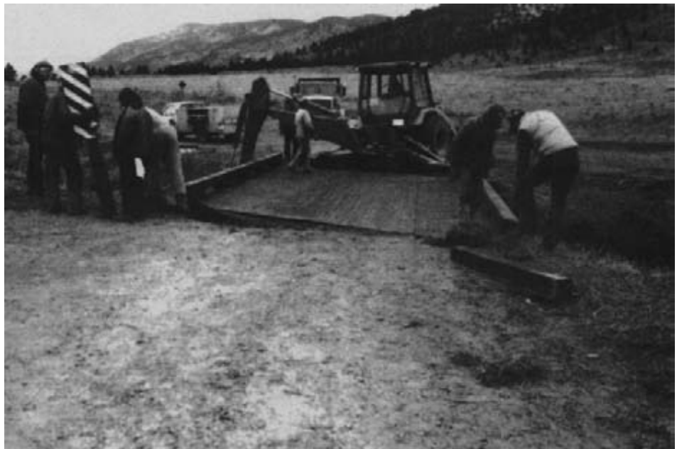
Figure 15-74. - Curbs are attached to the deck.
