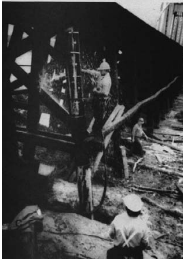
Figure 14-17. - Pile repair using pile restoration techniques (continued). (B) A replacement section is cut, and epoxy gel is applied to the contact surfaces. (C) The replacement section is placed and banded to the existing pile (photos courtesy of Osmose Wood Preserving, Inc.).
