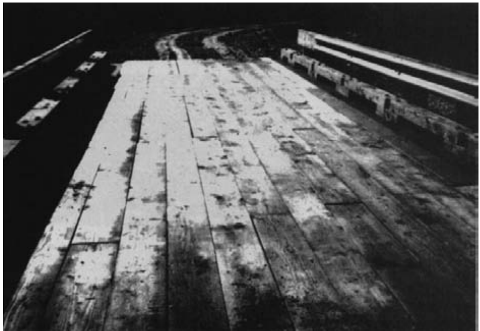
Figure 11-12. - Typical lumber wearing surface.
