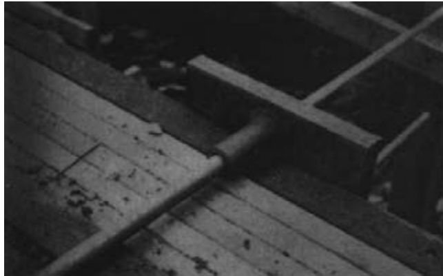
Figure 15-40. - Prestressing anchorage used at the Pickerel River Bridge.
