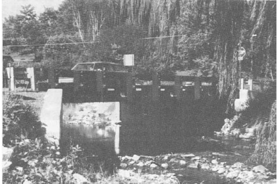
Figure 2-28- Stress-laminated deck bridge built near State College, Pennsylvania, in 1987. The bridge is 28 feet wide and was constructed from 4-inch-wide by 16-inch-deep lumber laminations.
