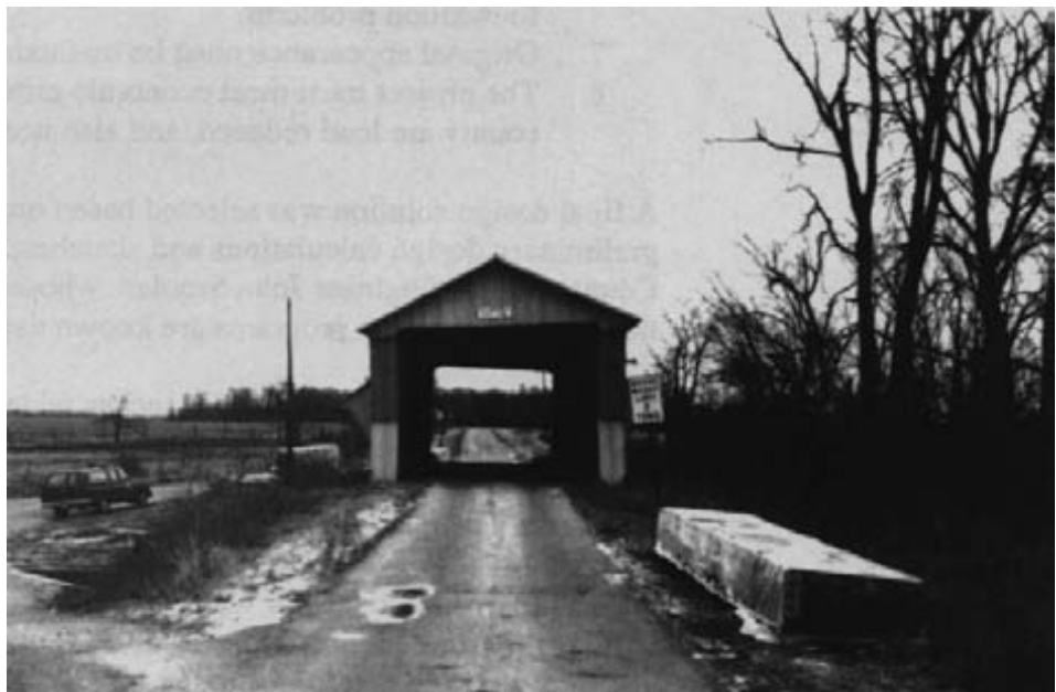
Figure 15-27. - Covered bridge on Winget Road before rehabilitation work began. Note the excessive rack and twist of the truss.
