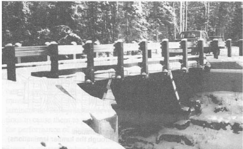
Figure 2-29.- Stress-laminated deck bridge with stress-laminated slant-leg supports, built near Espanola, Ontario, Canada, in 1981. The bridge spans approximately 55 feet and supports two traffic lanes (photo courtesy of the Ontario Ministry of Transportation).
