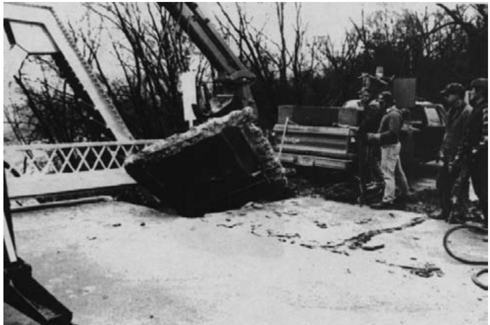
Figure 15-48. - The concrete deck was removed in approximately 5-foot-square sections by the Sauk County Highway maintenance crew. The concrete was broken using jackhammers, and reinforcing bars were flame cut. The sections were lifted and loaded on the trucks with a hydraulic excavator.
