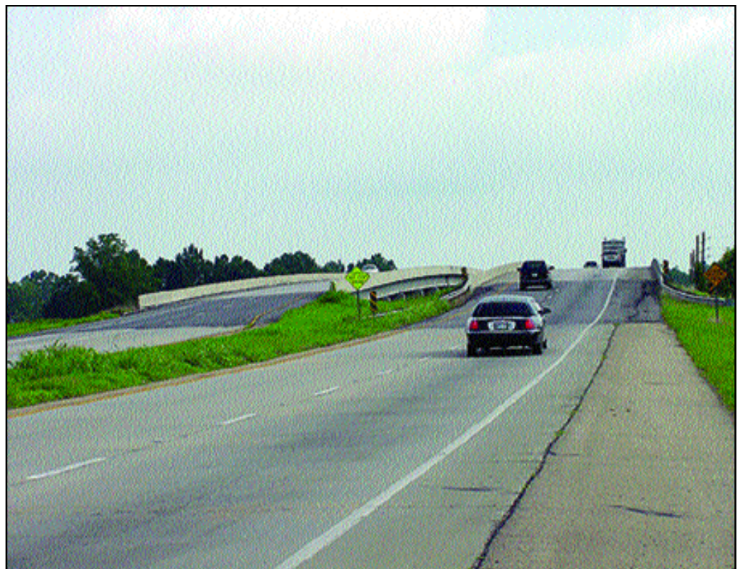
Corrective overlay on deflected approach slab
