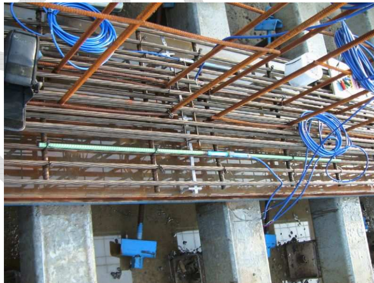
Figure A-2 Sisterbar installed next to a prestressing strand at midspan.
