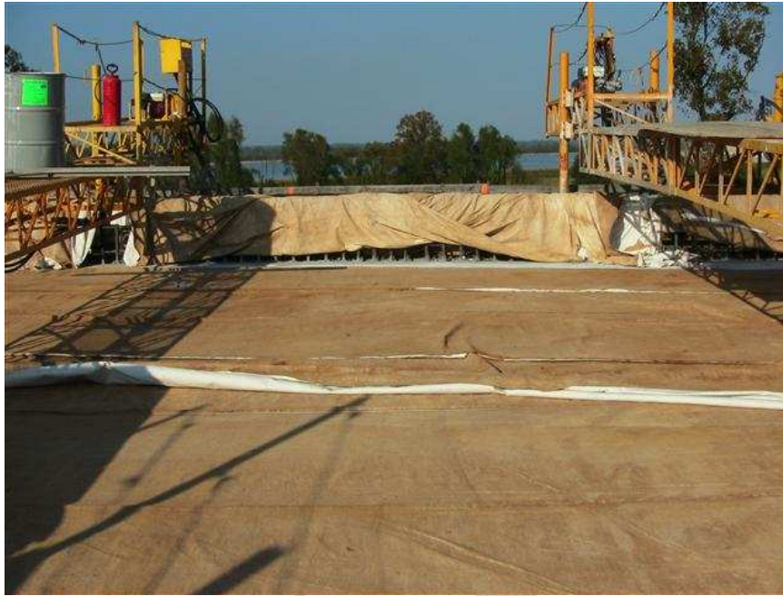
Figure A-13 Curing of bridge deck.
