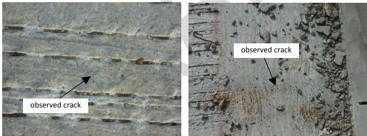
(a) in the middle of deck (skewed)
