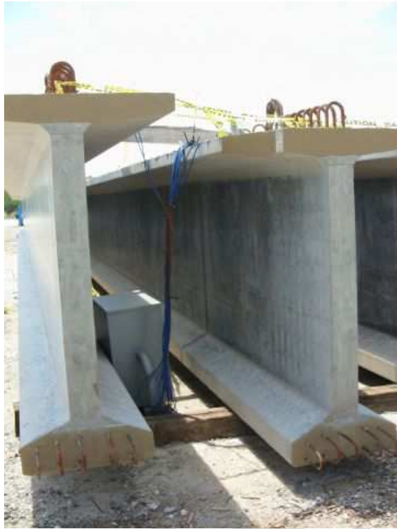
Figure A-11 Datalogger location while monitoring of curing girders in casting yard.
