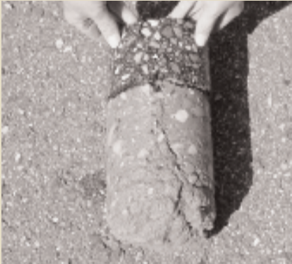
Figure 2 Reflection crack, not covered by warranty provisions
