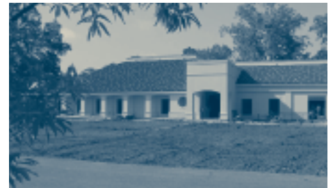
Back view of TTEC as of May 2005
