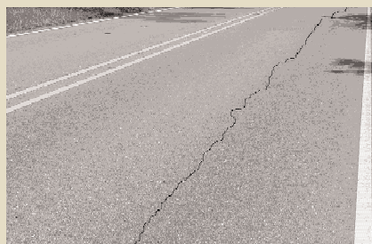
Figure 1 Cracks exceeding warranty requirements (retouched for better visibility)
