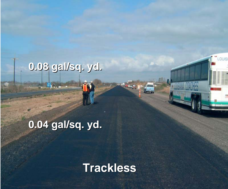
0.08 gal/sq. yd. SS-1 Uniformly distributed???
