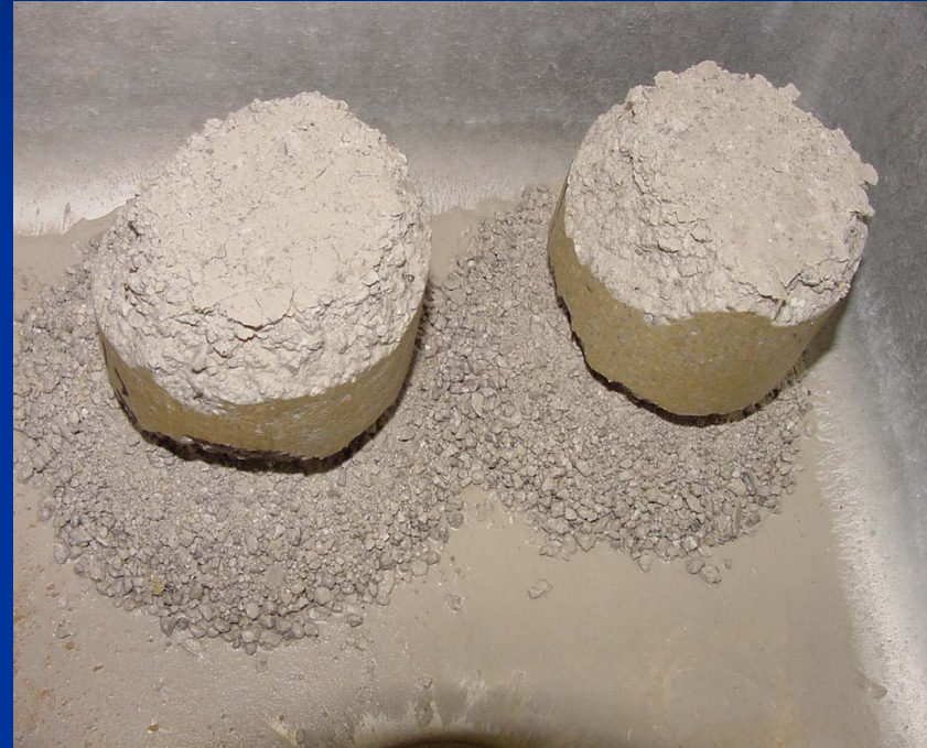
Dramatic deterioration of strength
