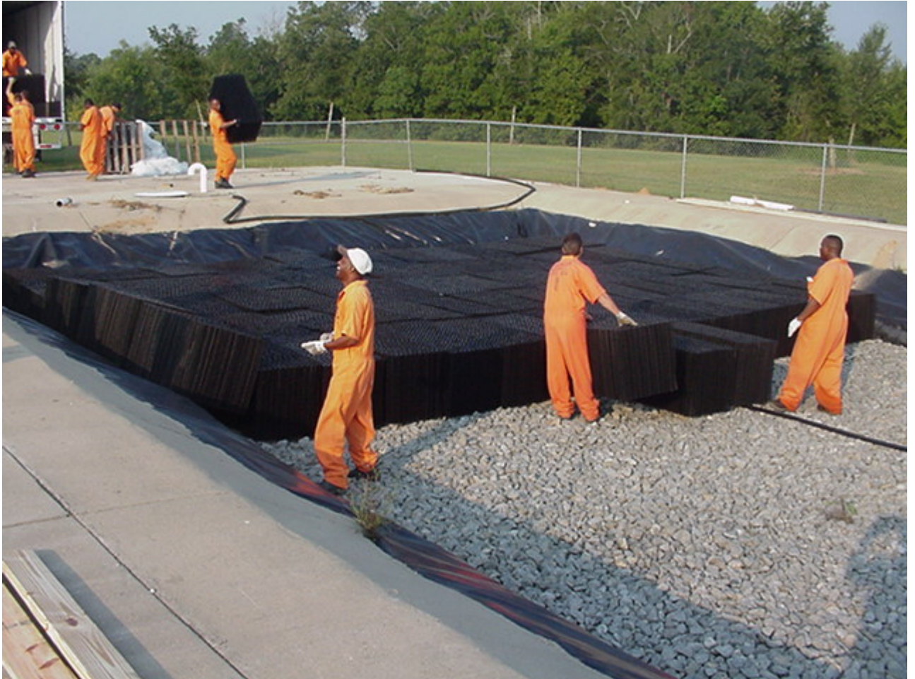
Figure 4 Placement of synthetic media – cell 3
