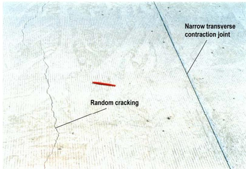
(a) Random crack propagated in the concrete slab about 3 ft. from the early entry dry cut contraction joint
