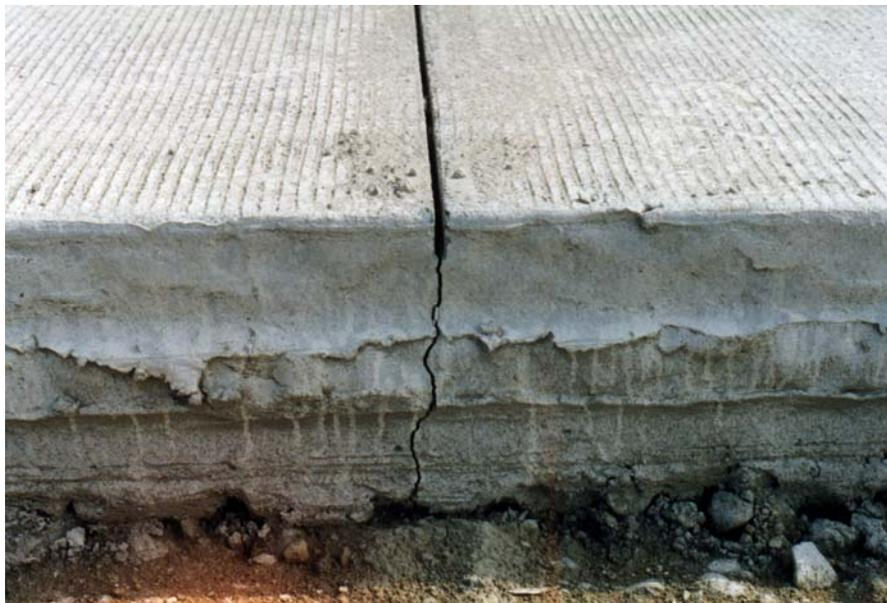
(b) Controlled crack developed underneath the narrow transverse contraction joint at test section S2 established using the early entry dry saw cut method
