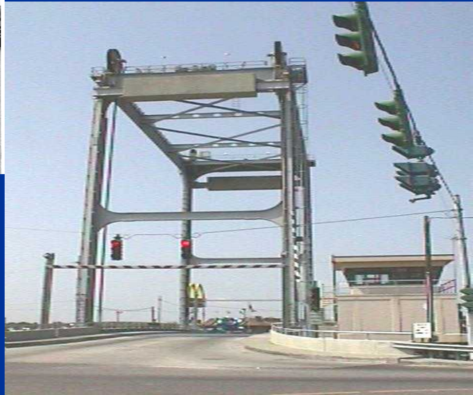
STEEL TOWERS - BAYOU LAFOURCHE AT CUTOFF
