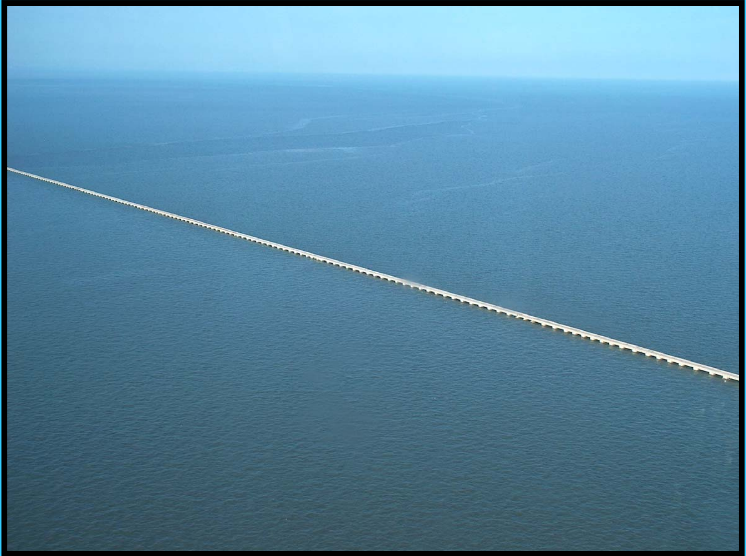
THE NORTH SHORE R.R. BRIDGE
