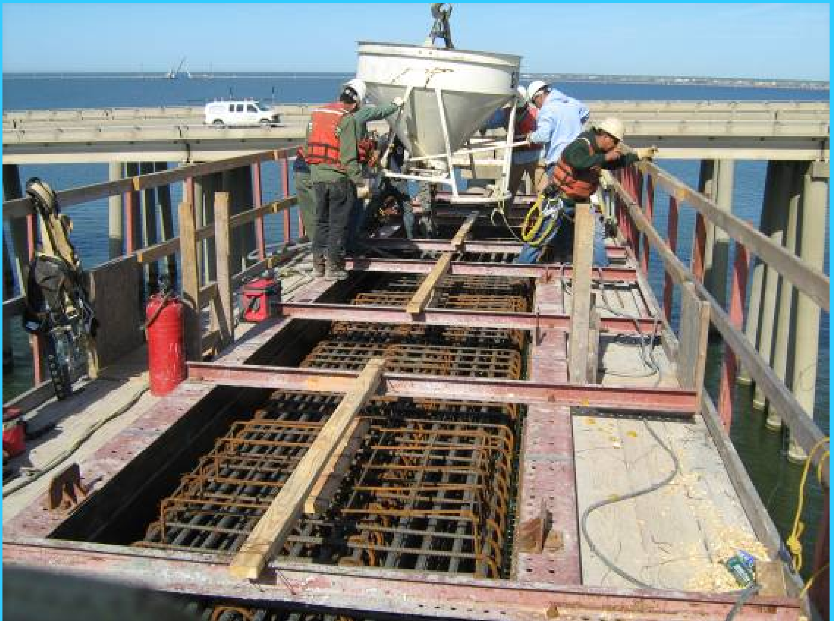
Placing Concrete for the Pier Cap at M-16 Westbound.
