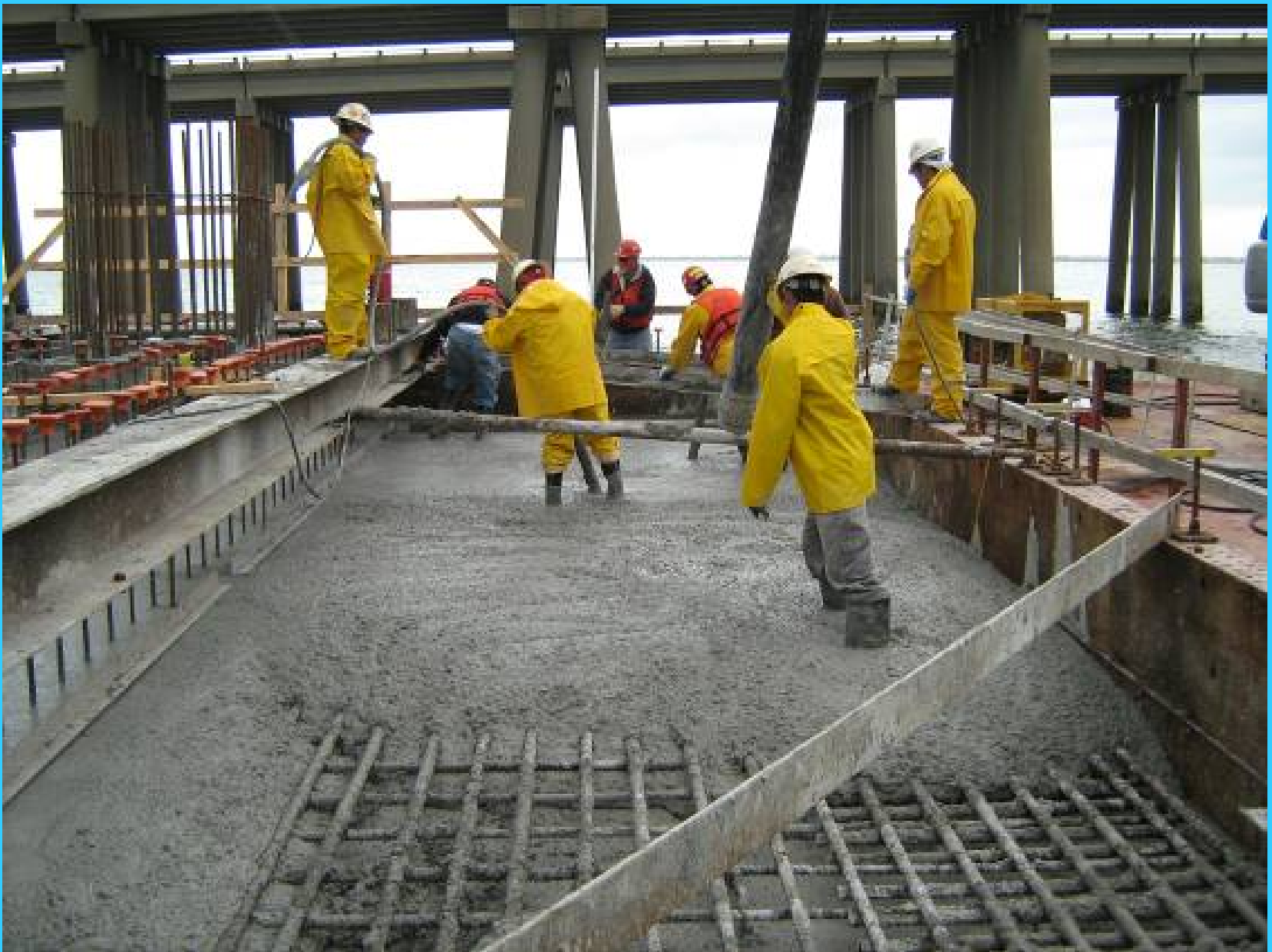
Placing Concrete for the Footing at M-13 Westbound.
