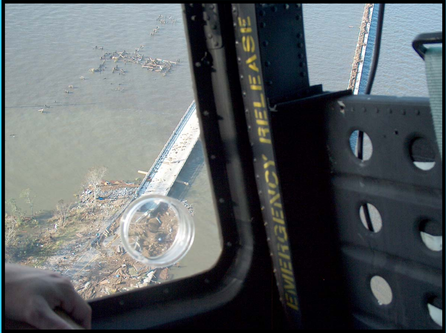
THE NORTH SHORE US 11 BRIDGE
