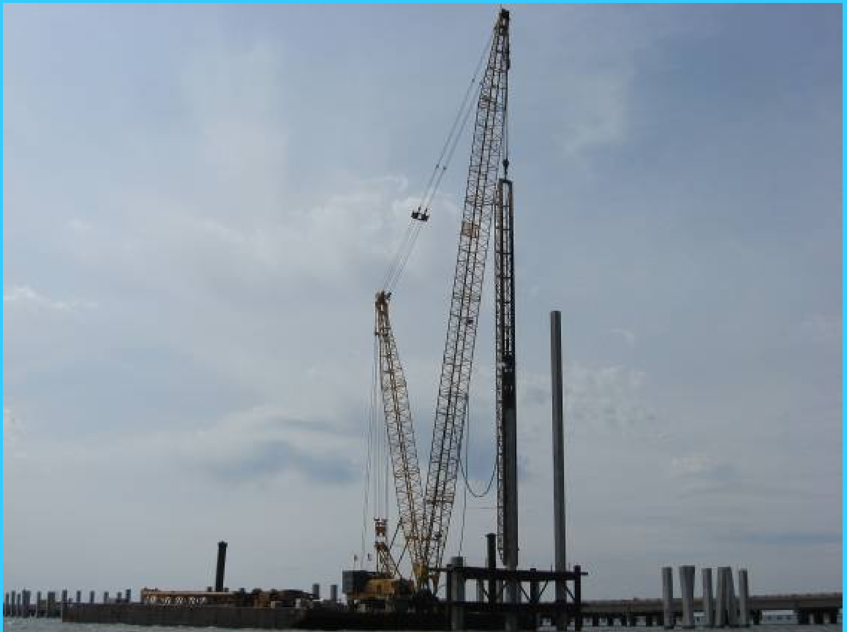
Driving 36" Pile at Bent S-81 Eastbound.
