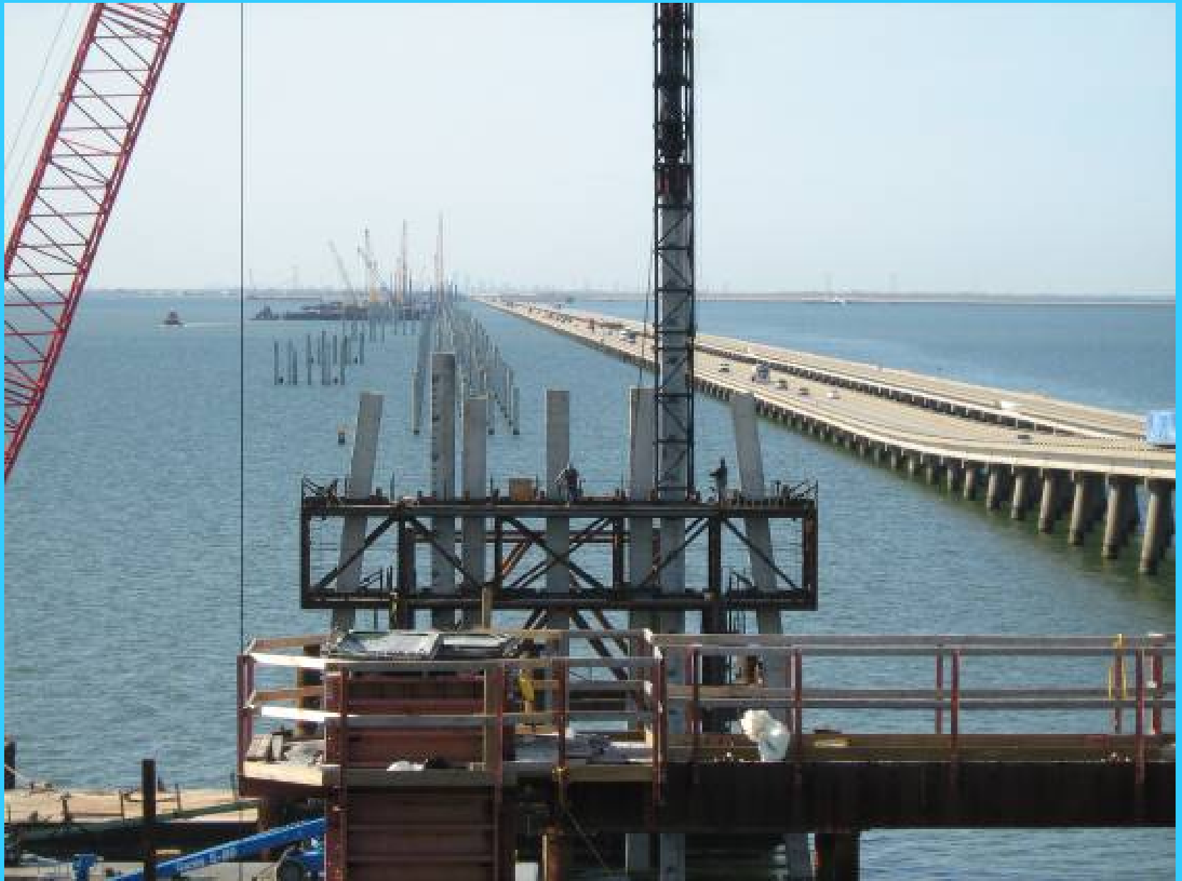
Driving 36" Pile at Bent M-12 Westbound.
