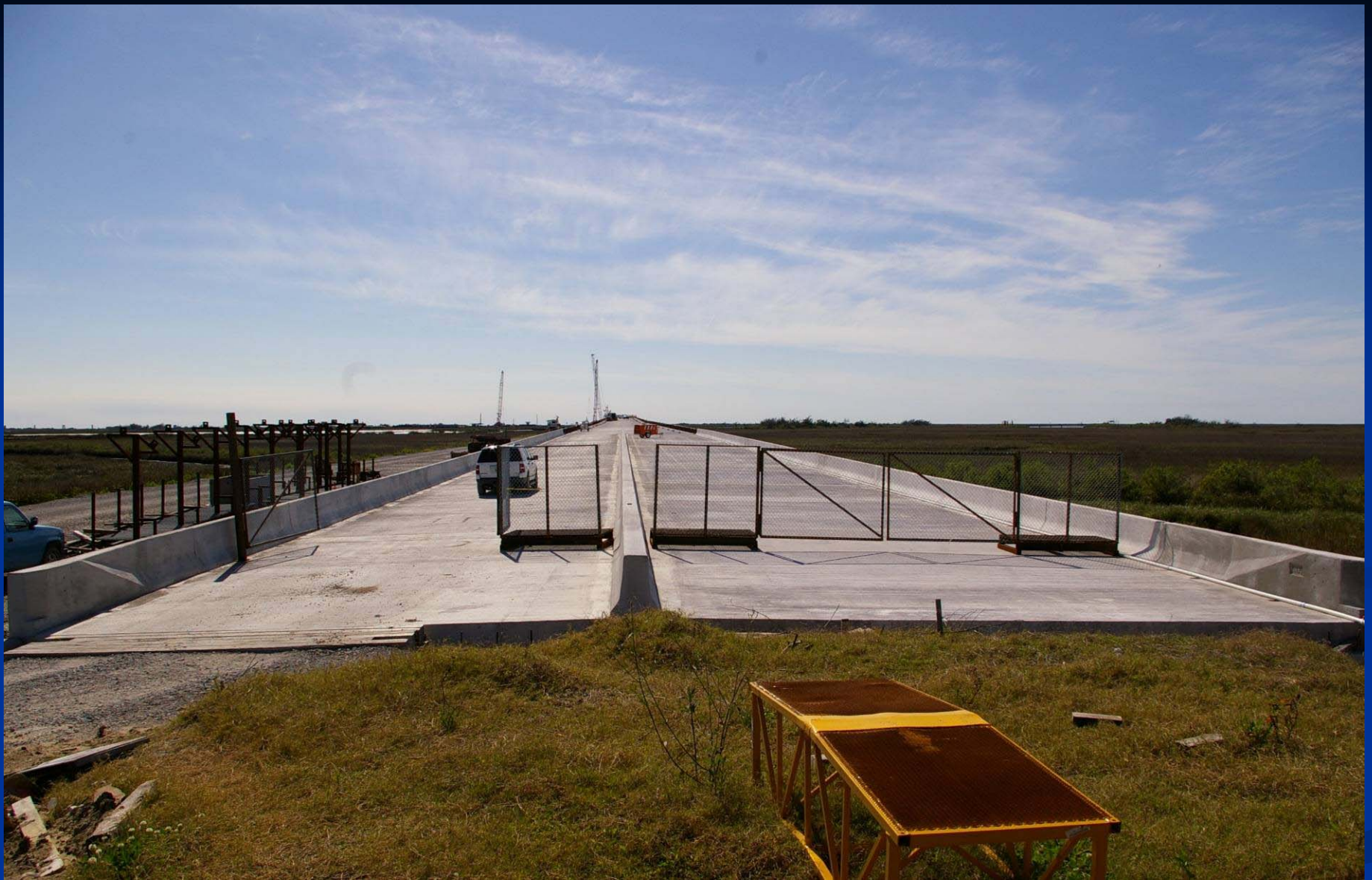
North Connector in area of ORT plaza (February 2008)
