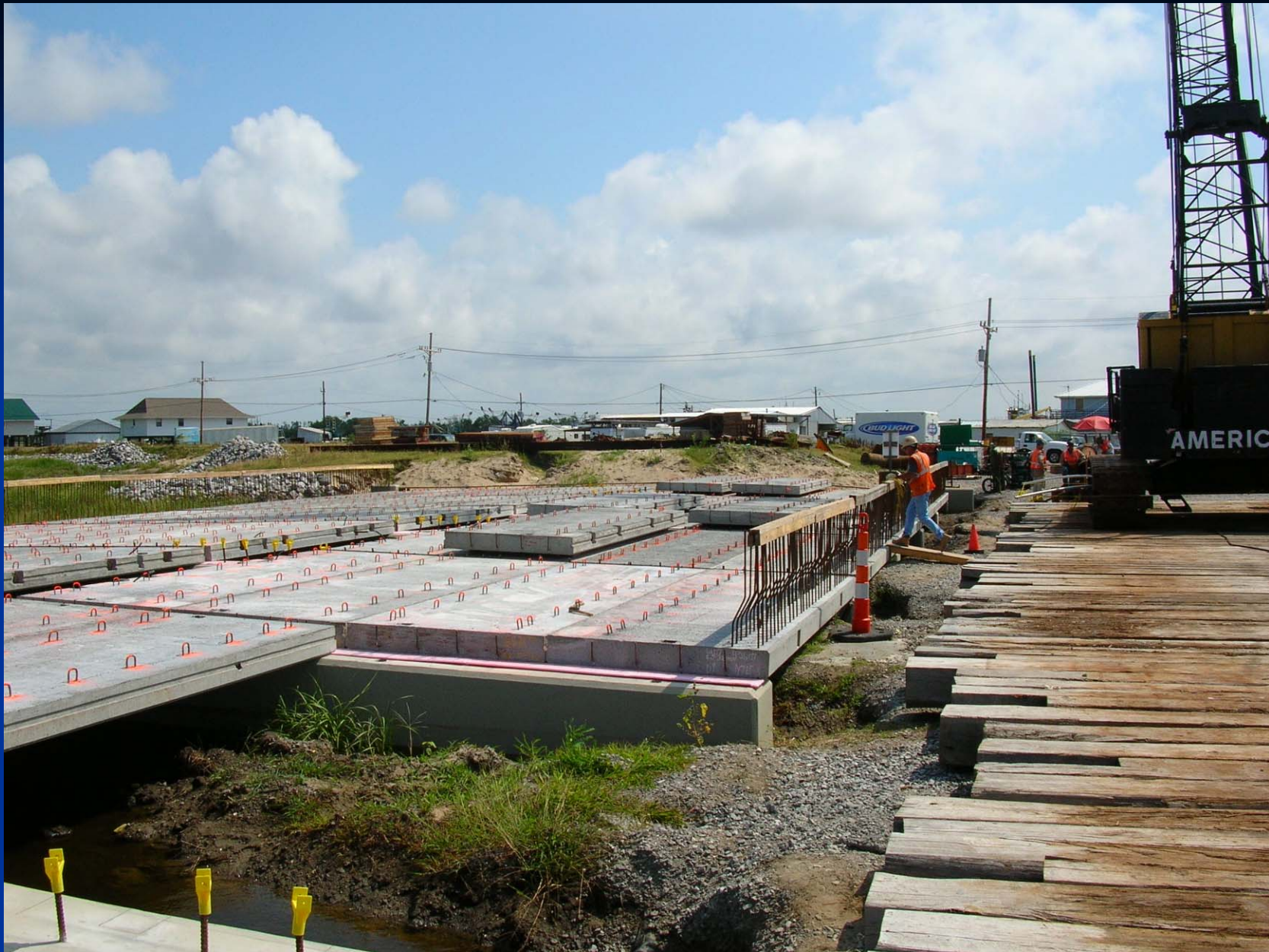
VE 'd Precast Slab Units on Connectors
