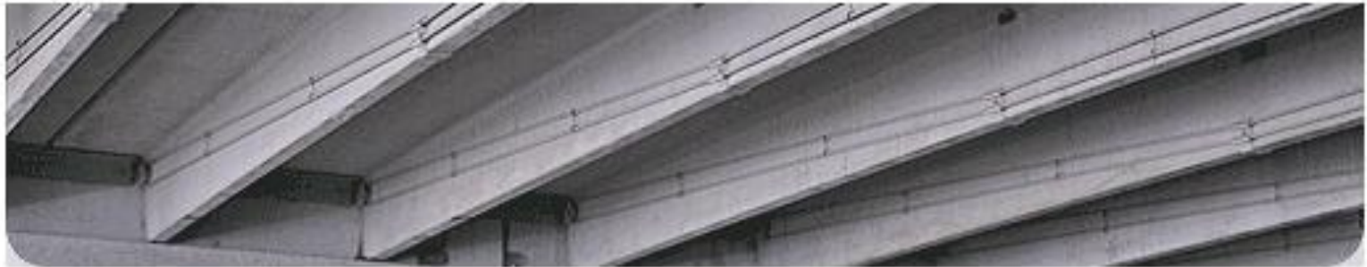
Strengthening with External Post-Tensioning
