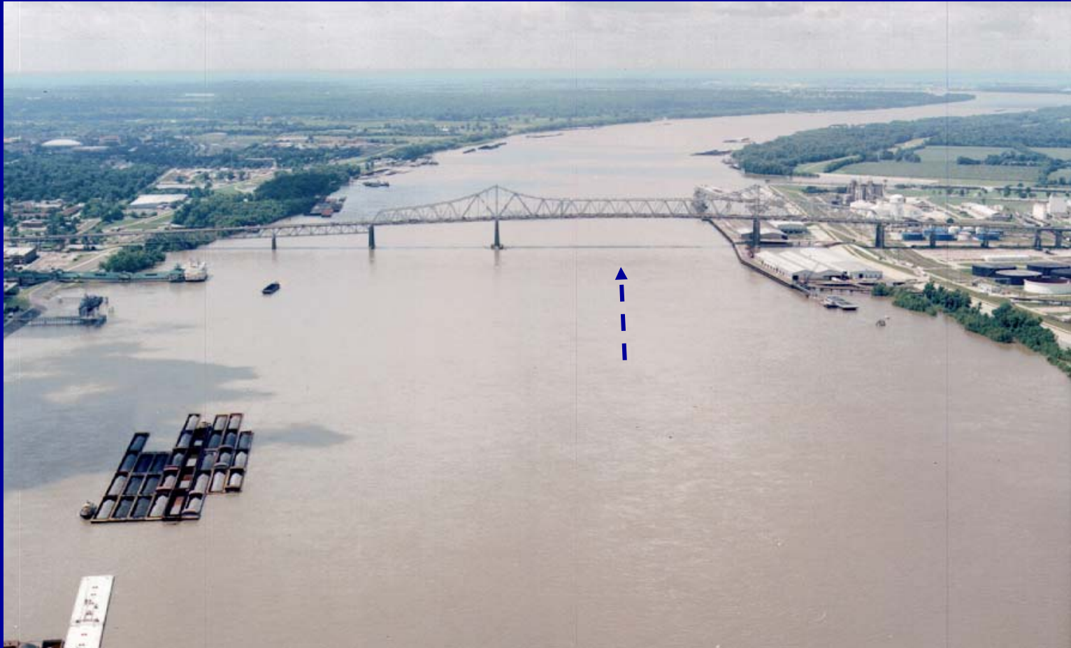
Bridge View Looking Downstream
