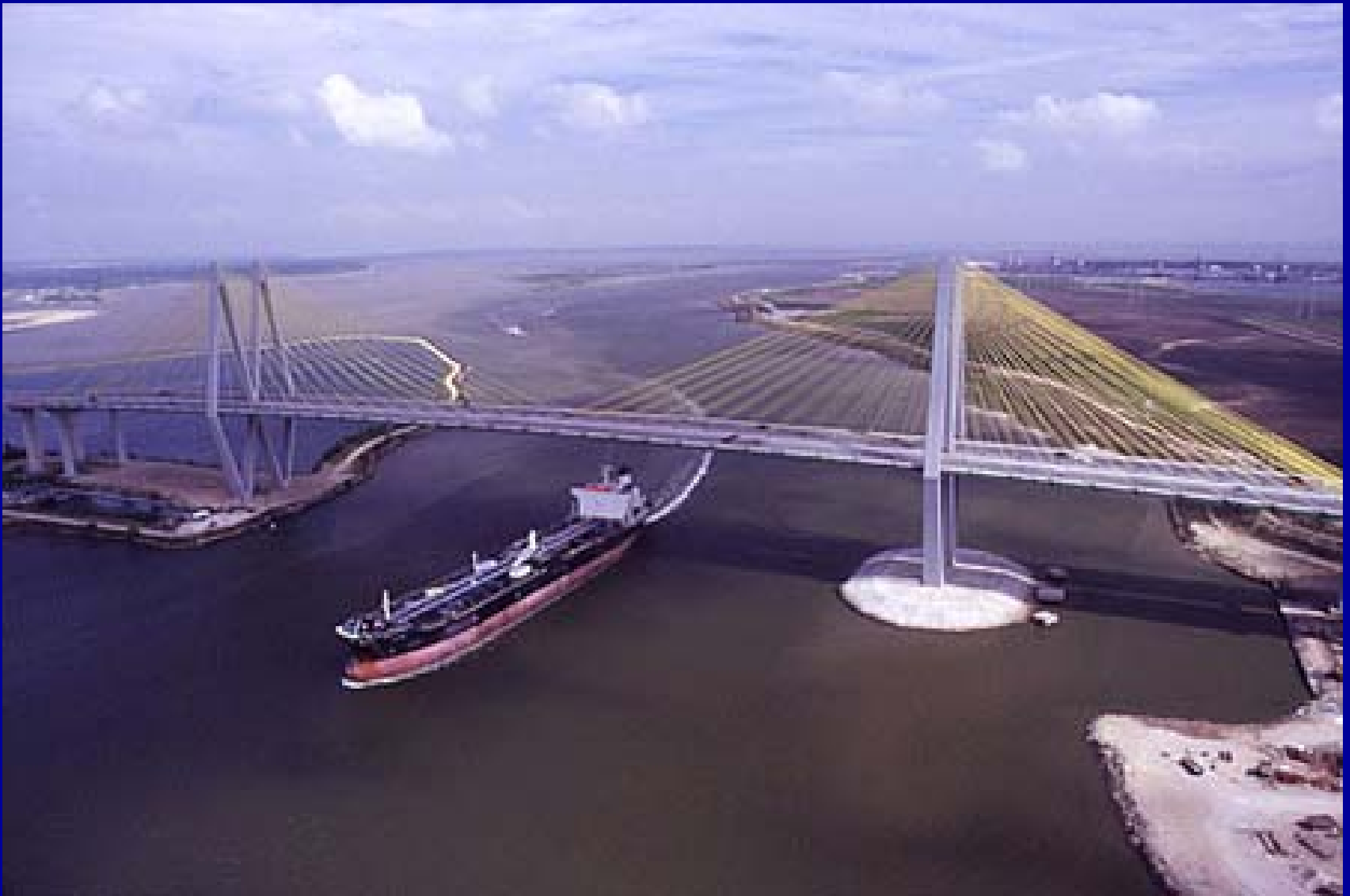
Fred Hartman Bridge, Houston Ship Channel
