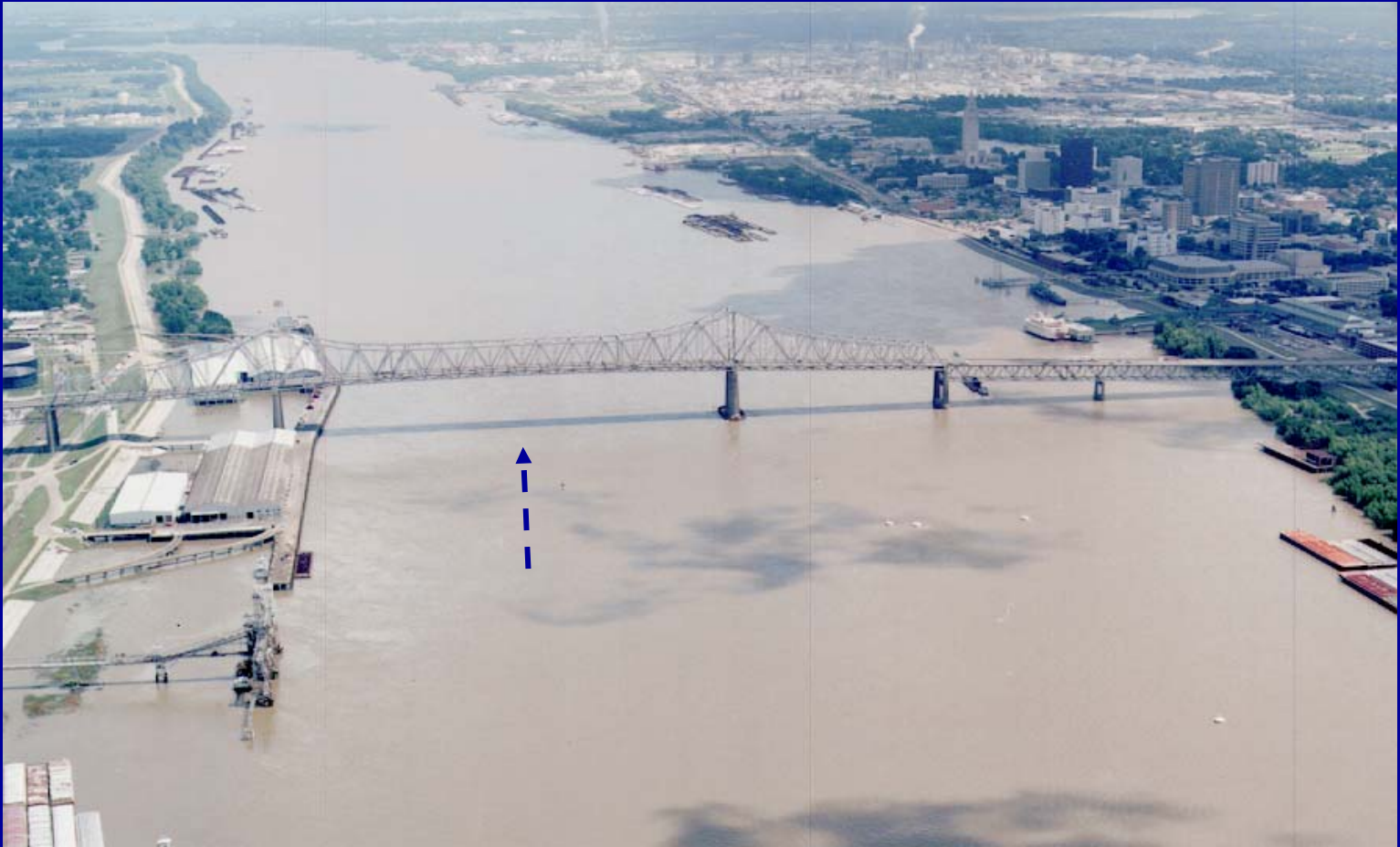
Bridge View Looking Upstream
