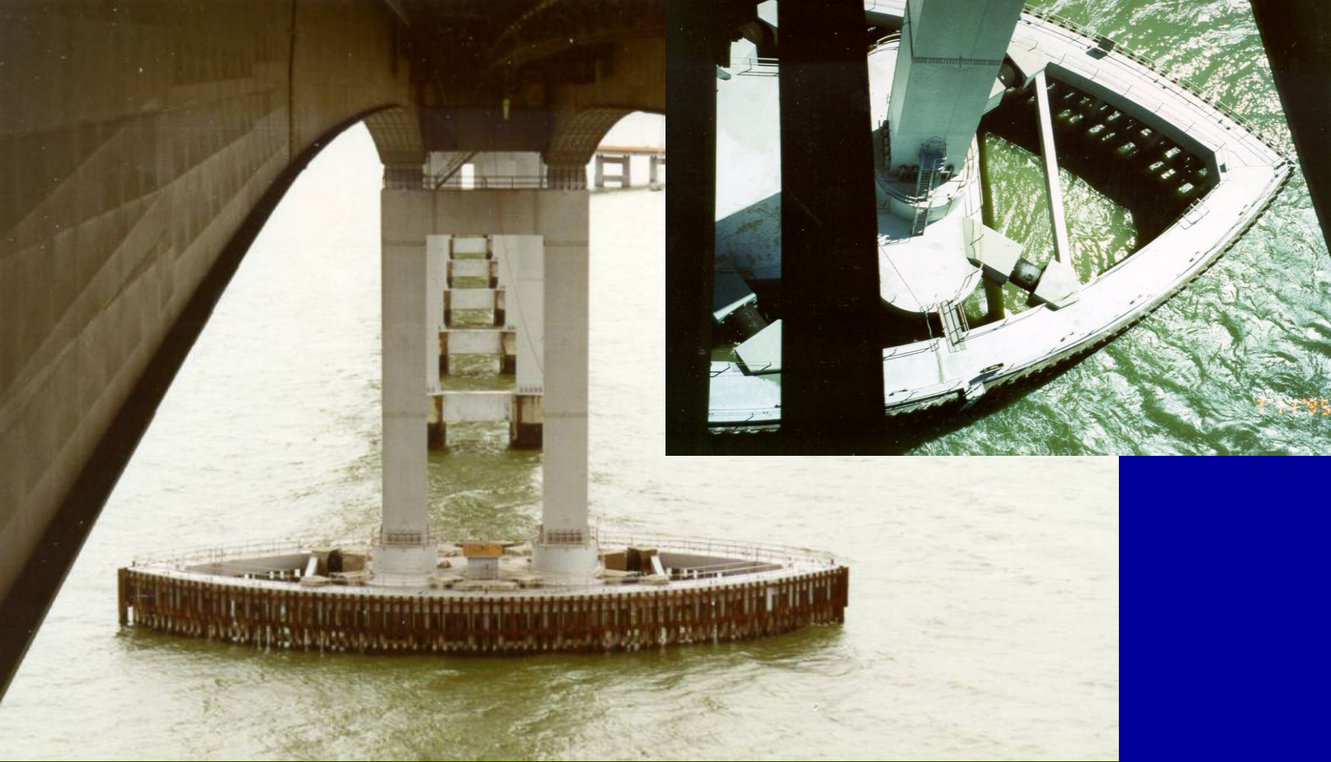
San Mateo Hayward Bridge, CA
