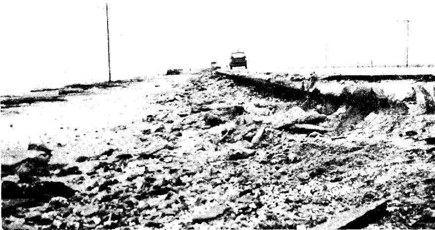
Figure 26. General Views of Damage to State Route 82 at Holly Beach, La. Caused by Storm of February 14, 1969. Damage such as this occurred for a distance of one mile on either side of the revetment tests.
