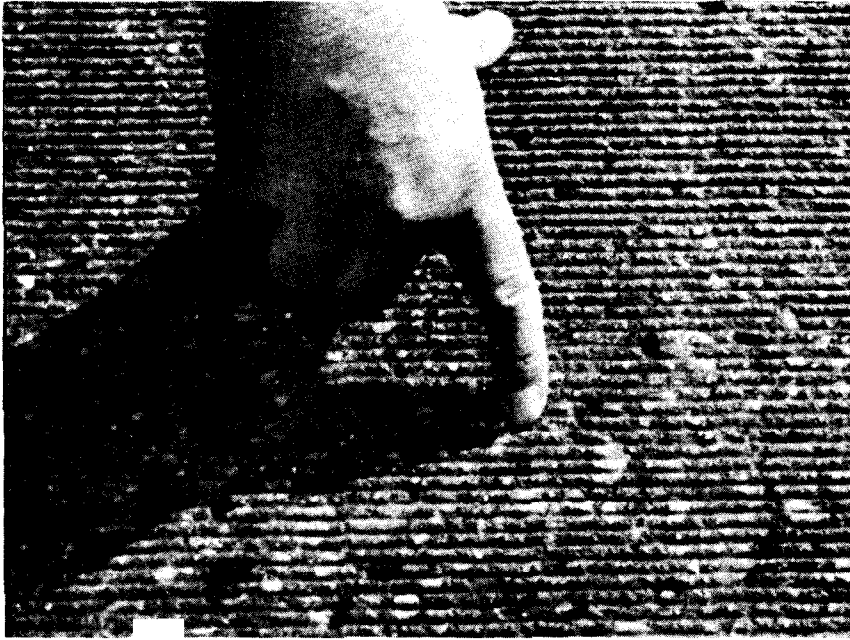
Figure 2: Grooved Pavement Before Traffic
