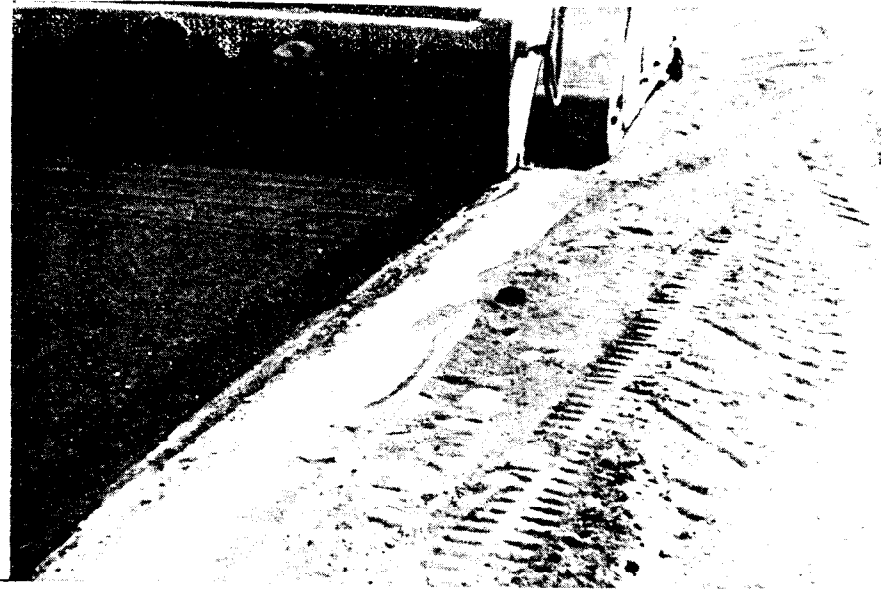
CEMENT LOSS DUE TO SPREADING BEYOND LIMITS OF BASE FIGURE 10a
