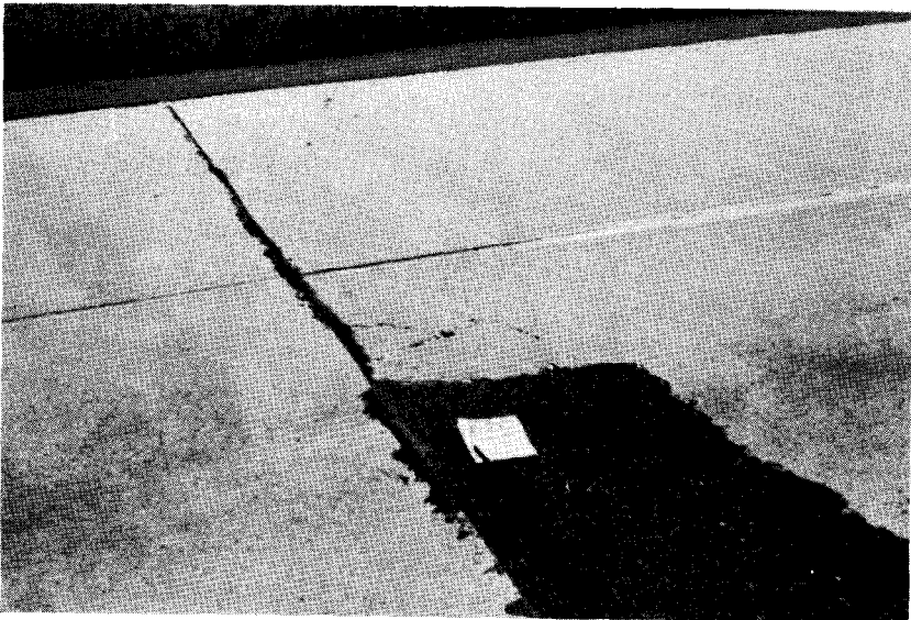
FIGURE 14 Asphalt Patch
