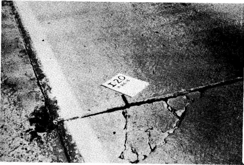
FIGURE 13 Corner Breakout
