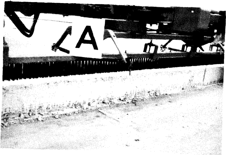
FIGURE 10 Heavy Polyplastic Broom on Transverse Texturing
