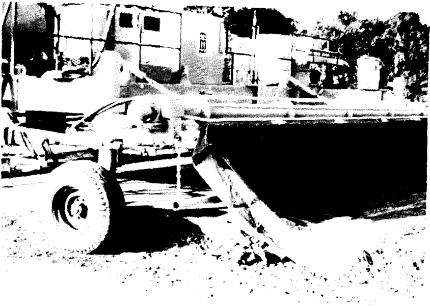
FIGURE 9 Normal Burlap Drag In Back of Float
