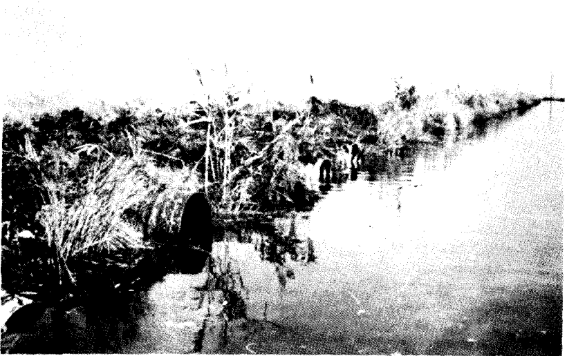
Typical Canal Installation (Location No. 10) FIGURE 3
