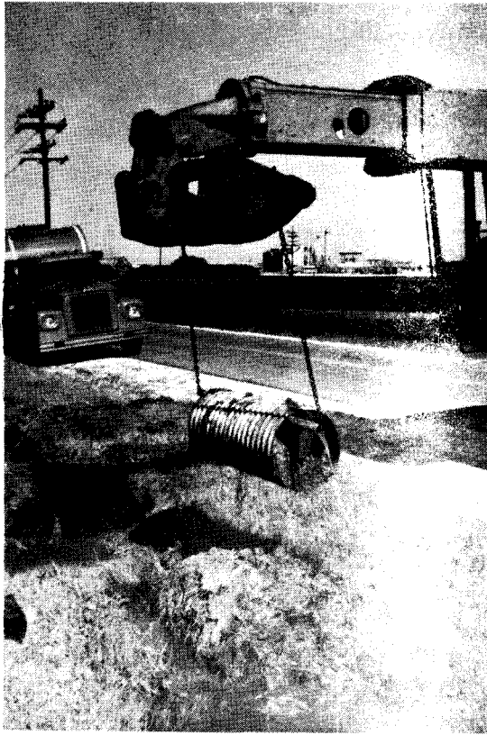
Drainage Pipe Removal FIGURE 4
