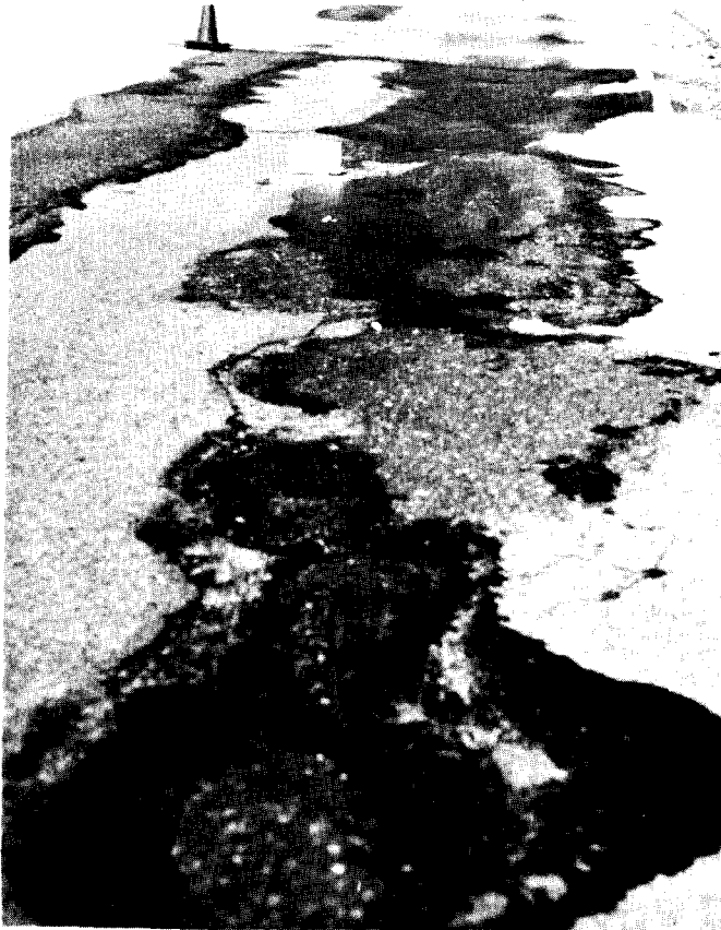
Figure 25 Overlay Patches Shoving on Span 8 (System 4)
