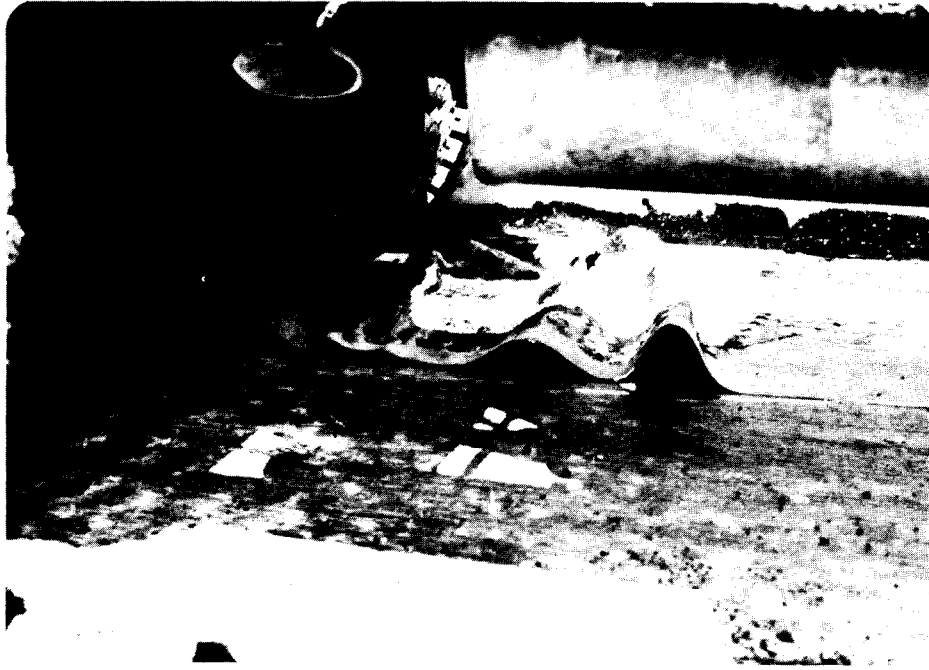
Figure 3 Truck Slides and Rolls Felt Paper from System 1 on Exit Ramp in Monroe
