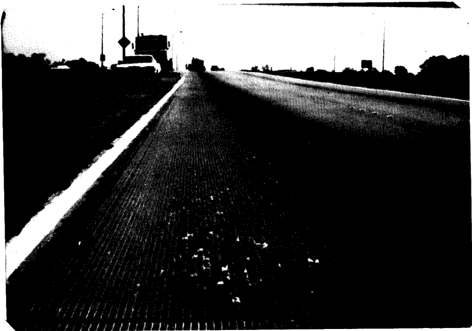
Spalled Grooves
