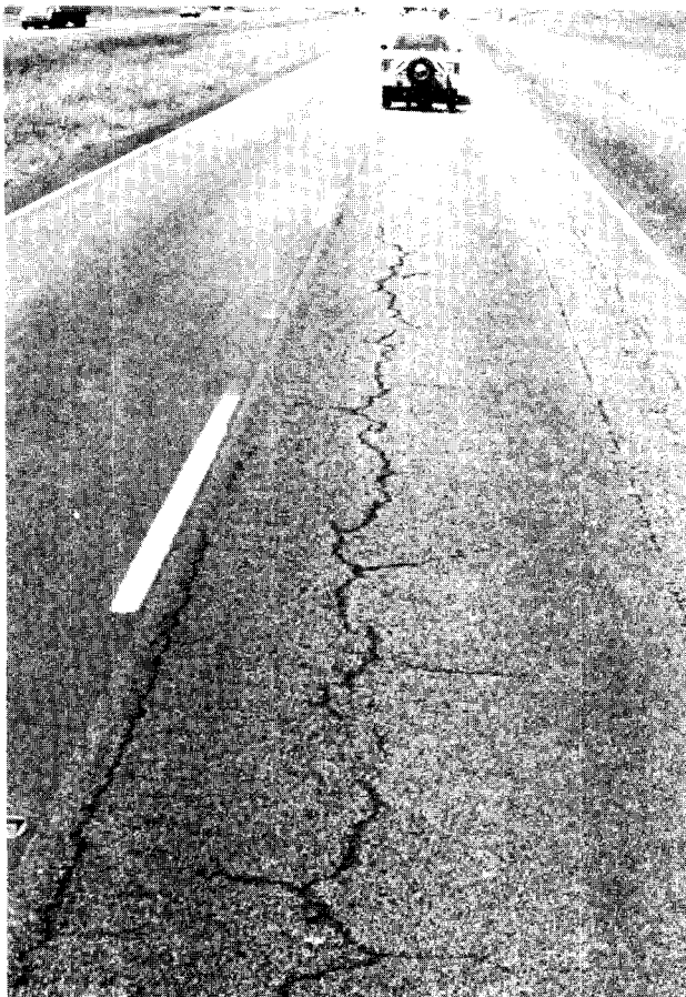
Wheelpath Cracking Reflecting Through Friction Course Figure 4
