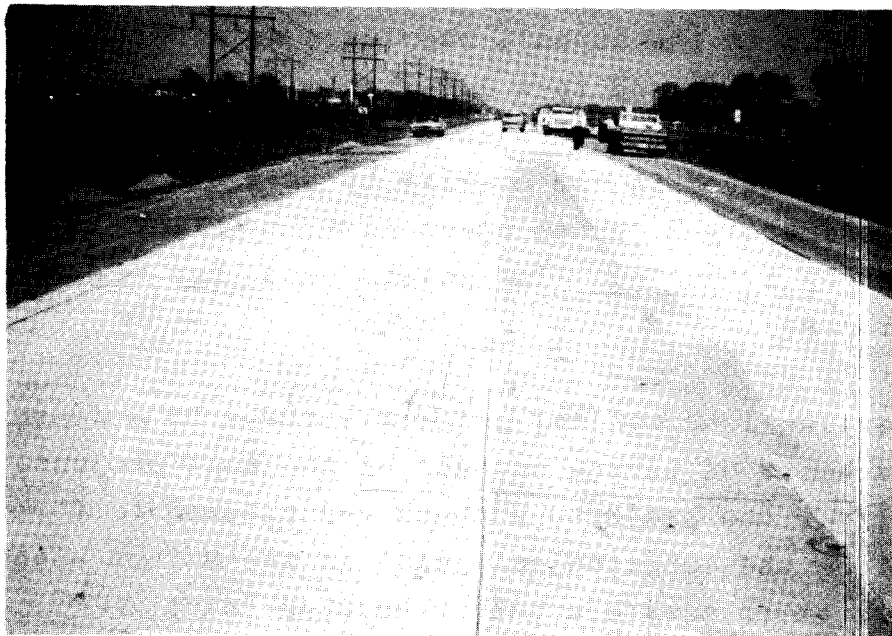
Cleaned Concrete Surface
