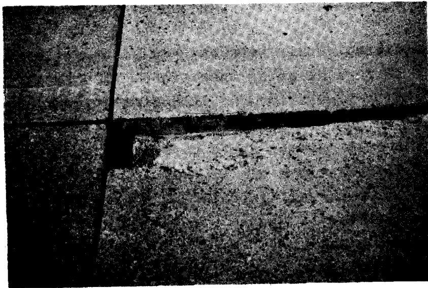
Concrete Removed Prior to Patching
