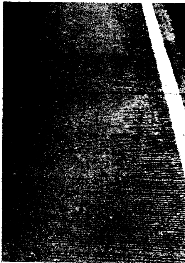
Wearing of Tined Finish in Wheel Paths
