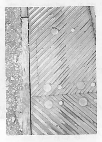
Indication of Internal Fracturing or Failure FIGURE 3 This type of failure was predominant in a similar GEN-TRAC II crossing at Patoutville, Louisiana. There are also many places where the rubber is delaminating from the steel substructure in the wheelpaths.
