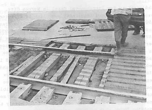
Broken Shim(s) and Excessive Pumping FIGURE 12
