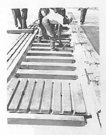
Aligning the New Replacement Gage Shims
