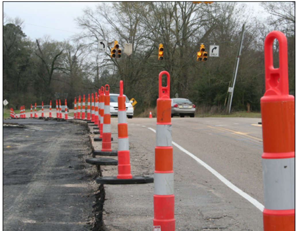
Construction Work Zone
