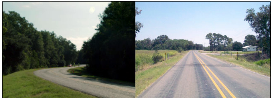
Figure 1. Two segments of Narrow Rural 2-lane highway in Louisiana
