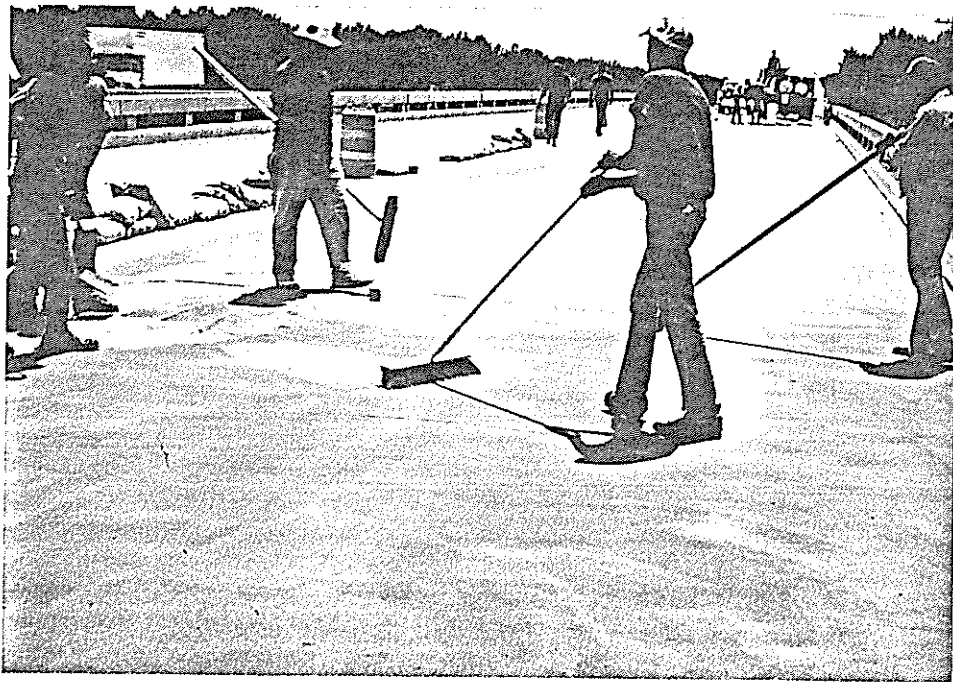
Sweeping the Excess Aggregate After the Final Coat
