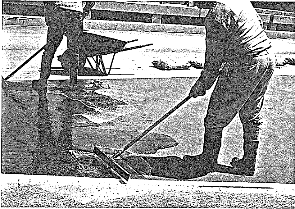
Spreading Dural Epoxy Over the First Lift
