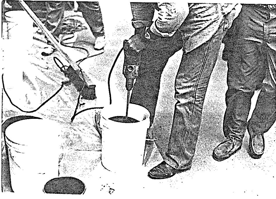
Mixing the Two Components of Epoxy
