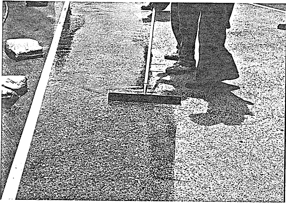
Spreading of the Epoxy (Dural)
