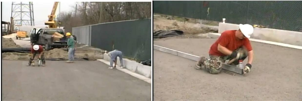
**Figure 12: Slab layout on base course**
