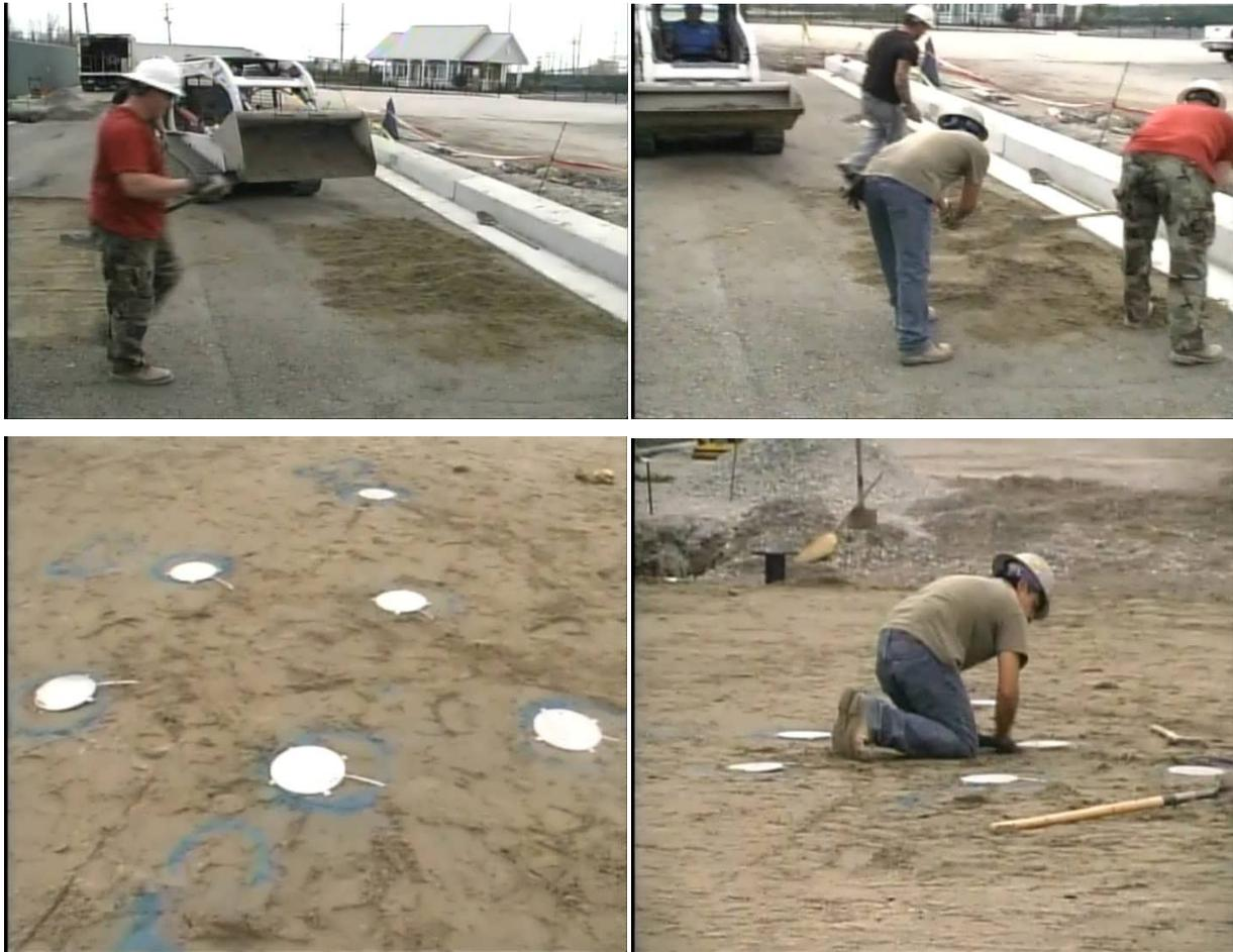
**Figure 13: Sand layer placement and sensors**
