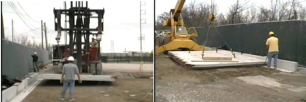
**Figure 14: Precast panel installation**
