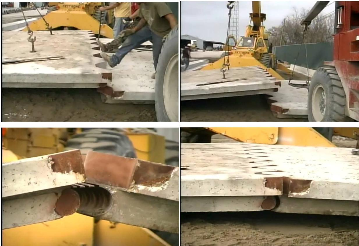
**Figure 15: Longitudinal joint stitching**
