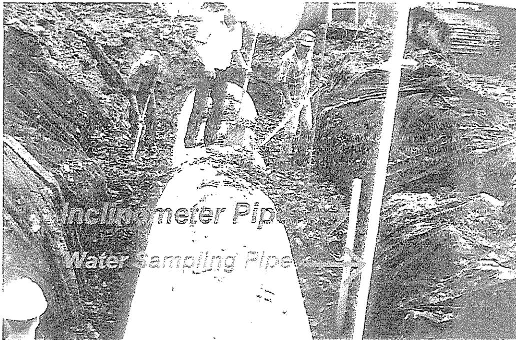
Figure 13. Installation of the vertical inclinometer in the field
