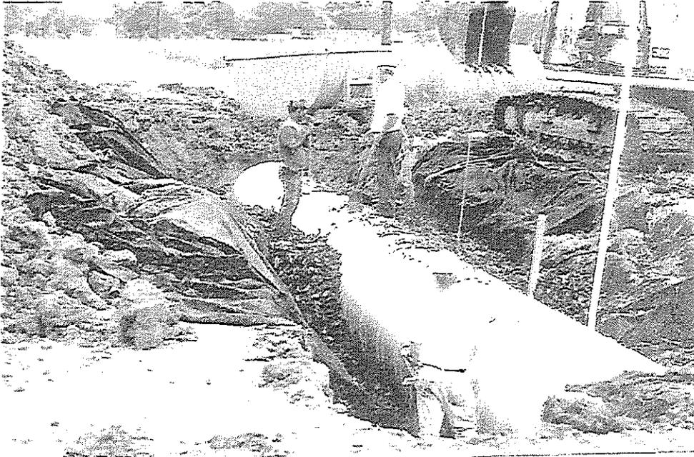
Figure 9. Placement of tire chips around the pipe
