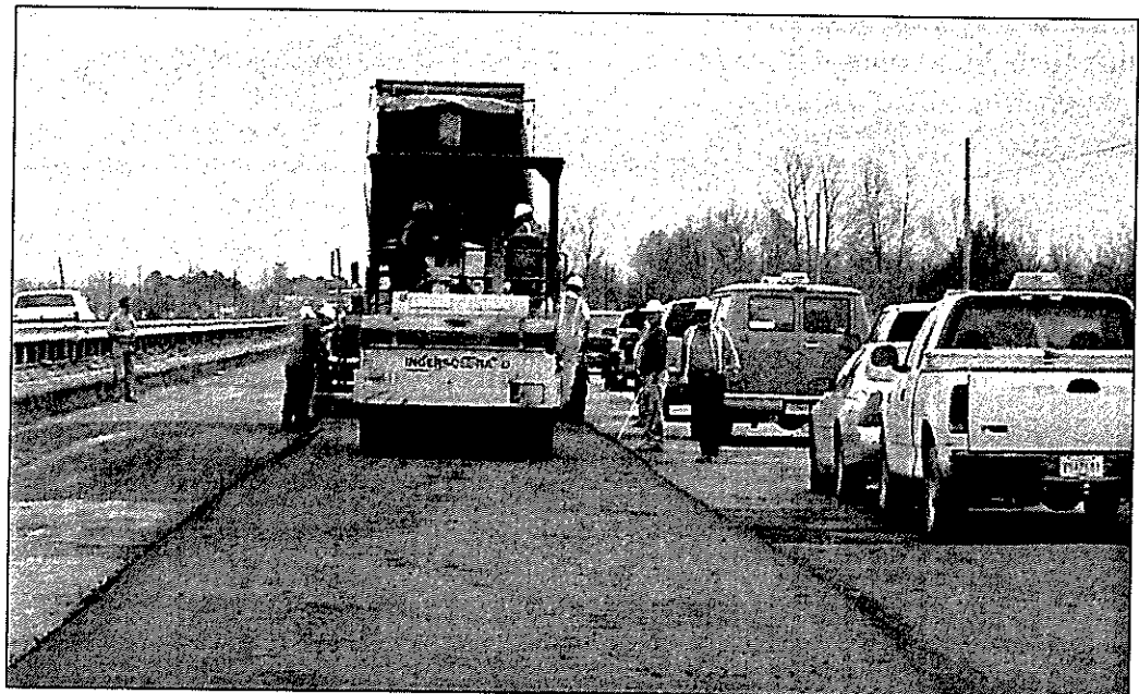
Asphalt pavement construction
