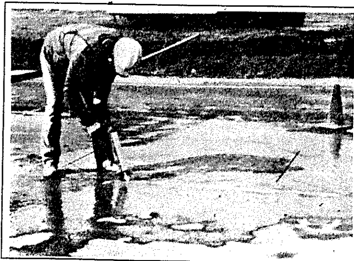
Loop failure resulting in unnecessary traffic delays and increased maintenance greatly affects the public.
