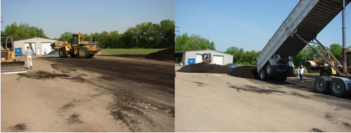
Figure 29 Placement of material by front-end loader and haul trucks
