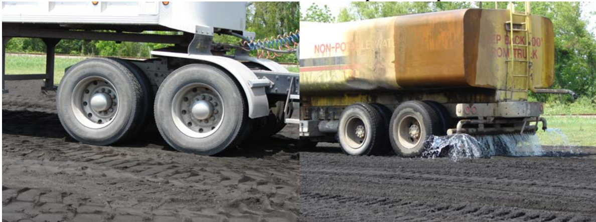
Figure 33 Haul truck and water trucks driving on the lifts with minimal rutting
