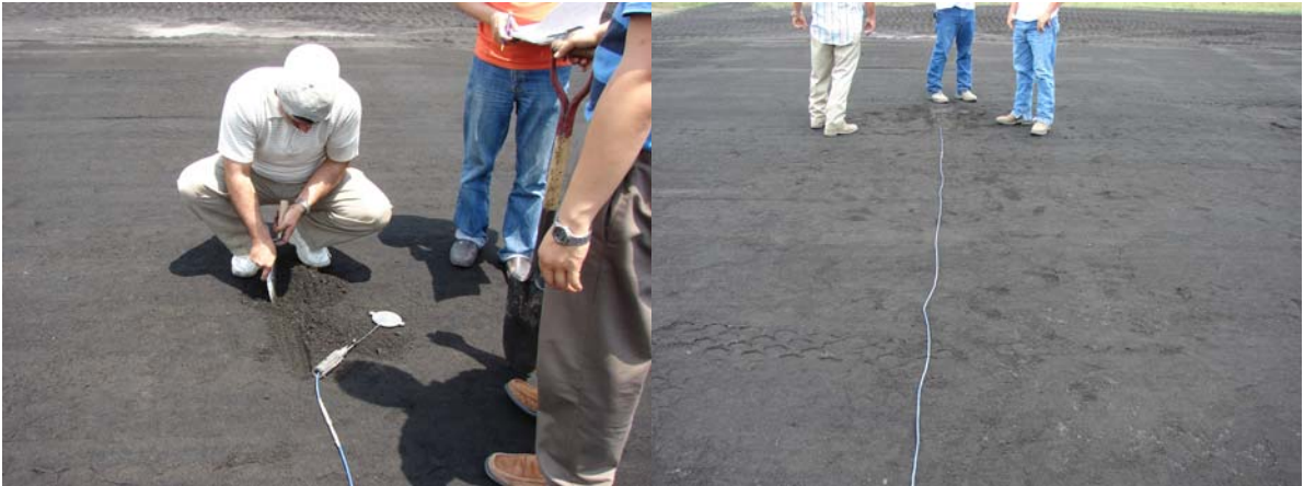
Figure 35 Pressure sensor and wire installation
