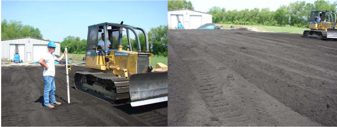
Figure 32 Laser level used to measure lifts and lifts prior to compaction
