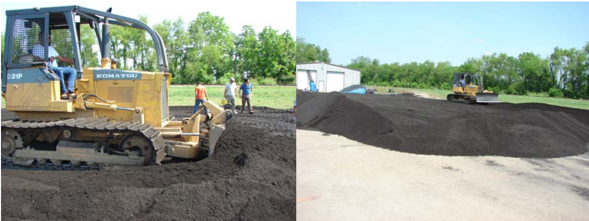
Figure 31 Komatsu D31P, dozer used to spread the bottom ash lifts
