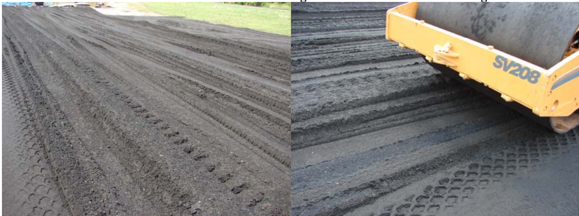
Figure 34 Before and after vibratory roller
