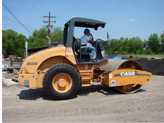
Figure 9 Case SV208, vibratory roller
