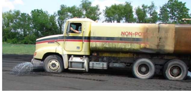
Figure 11 Water truck driver's wheel cut sharp
