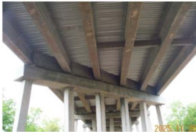
Figure 5 View of BNSF overpass
