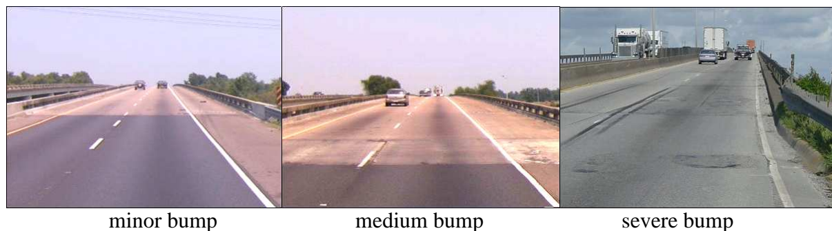
Figure 12 Bridge approach slabs
