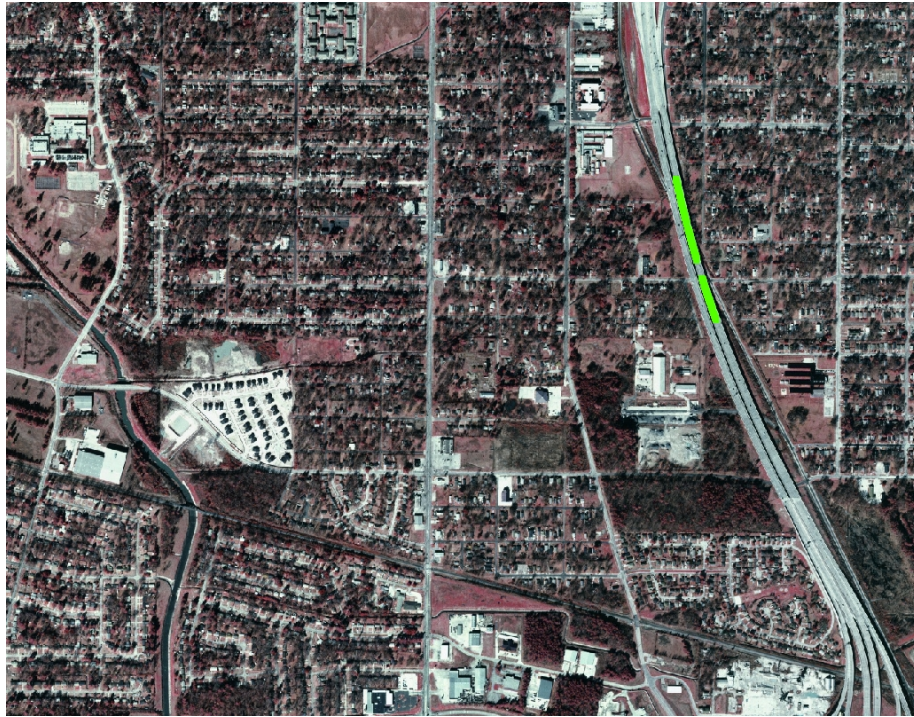
Figure 6 District 04 I-49 at Inner Loop
