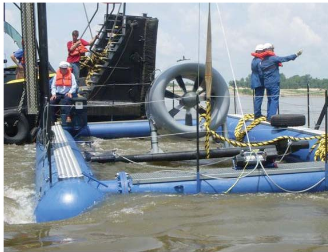
Figure 1 Deployment of a turbine
