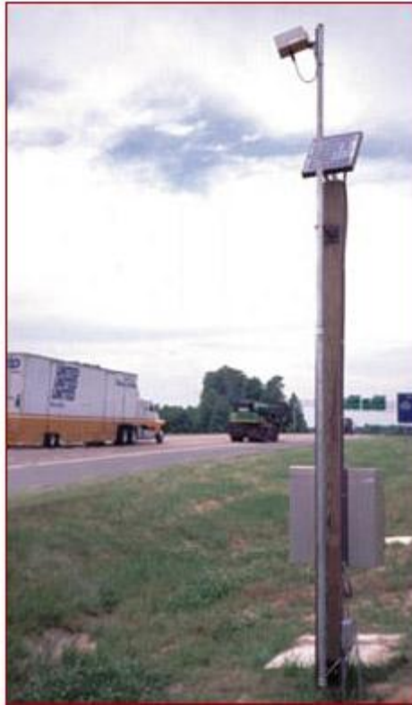
Figure 6 RTMS solar powered remote counting station
