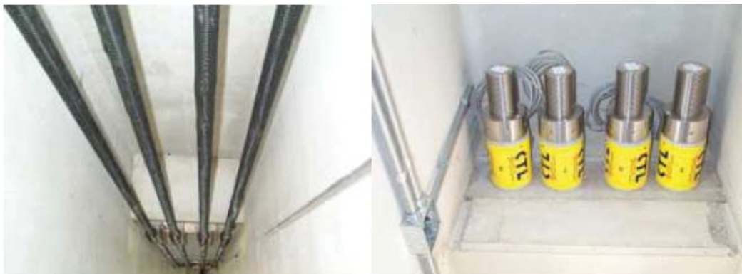
Longitudinal CFCC tendons and installed load cells
