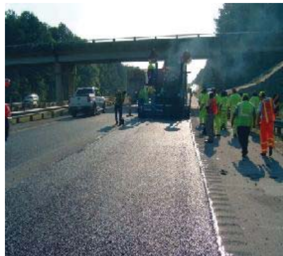
Figure 2 Workers laying down OGFC test sections
