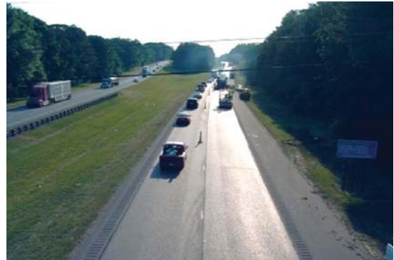
Figure 1 OGFC test section
