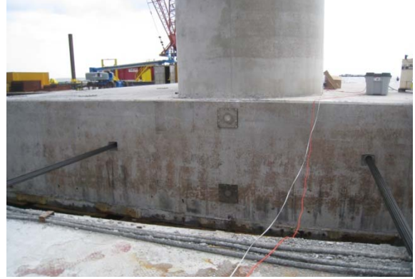
(b) E. Pier with steel strand tendons
