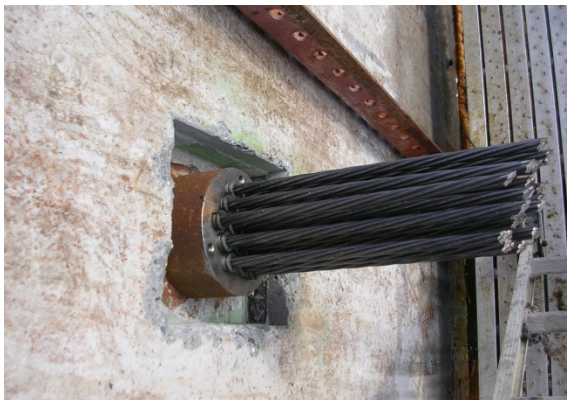
(c) Dead-end at the eastbound pier
