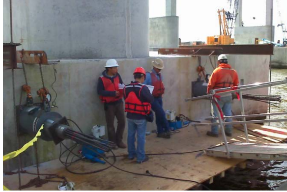
(a) Jacking system at the live-end of w. pier
