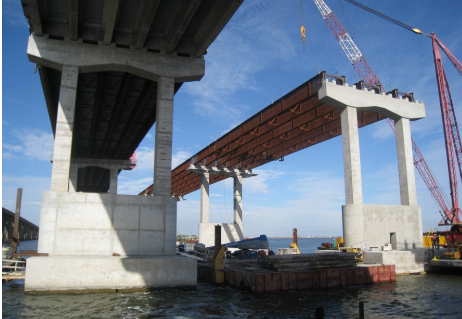
Figure 18 Load test site at M19 eastbound and westbound Piers
