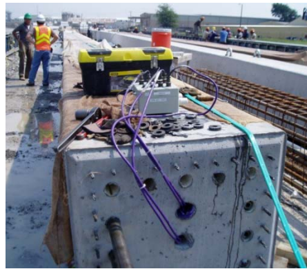
(b) Data Logger on Pile 1
