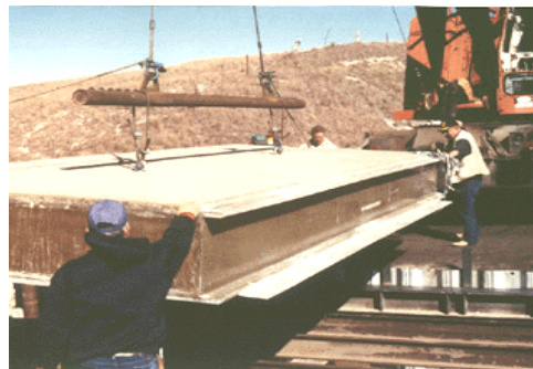
Figure 146 Installation of No-Name Creek Bridge, Russell, Kansas
