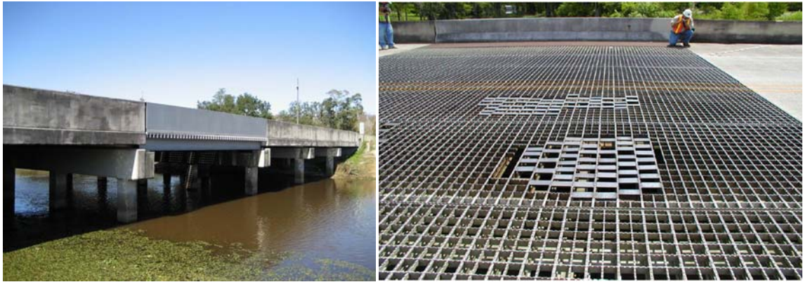
Figure 1 Pierre Part bridge
