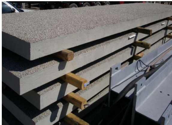
Figure 114 Finished bridge deck with non-skid surface
