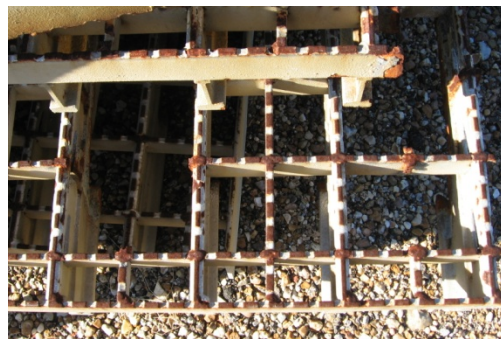
Figure 69 Lost sections in the steel bridge deck
