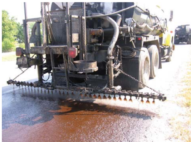
Figure 2-1 Application of Fog Seal on US-36 (Caltrans, 2009)
