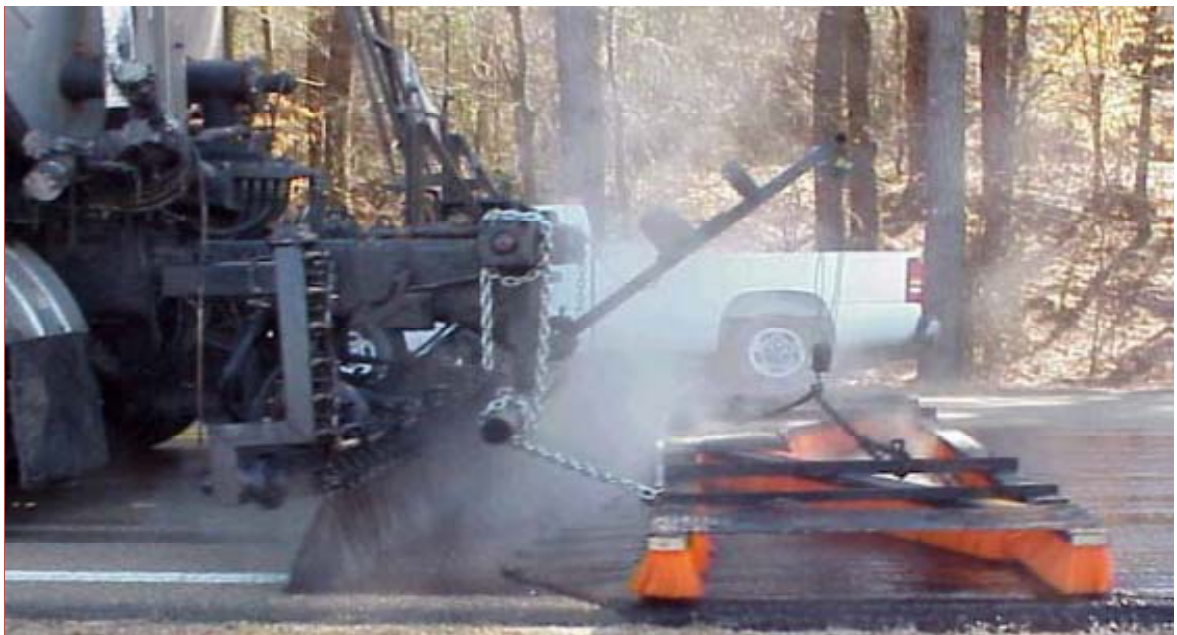
Figure 5-2 Application of Scrub Seal (Howard, 2009)
