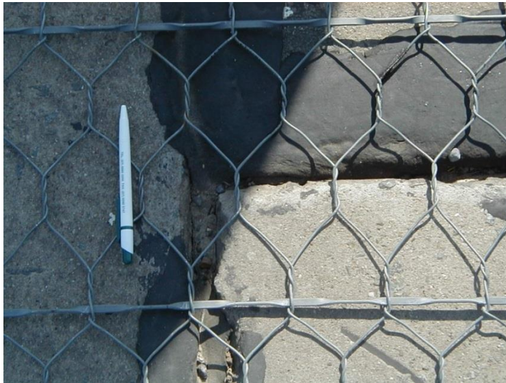
Figure 32 Steel reinforcing mesh [85]
