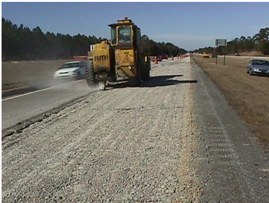
Figure 26 Rubblized concrete pavement [63]
