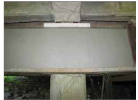
Pile cap repaired with high-strength composites.
