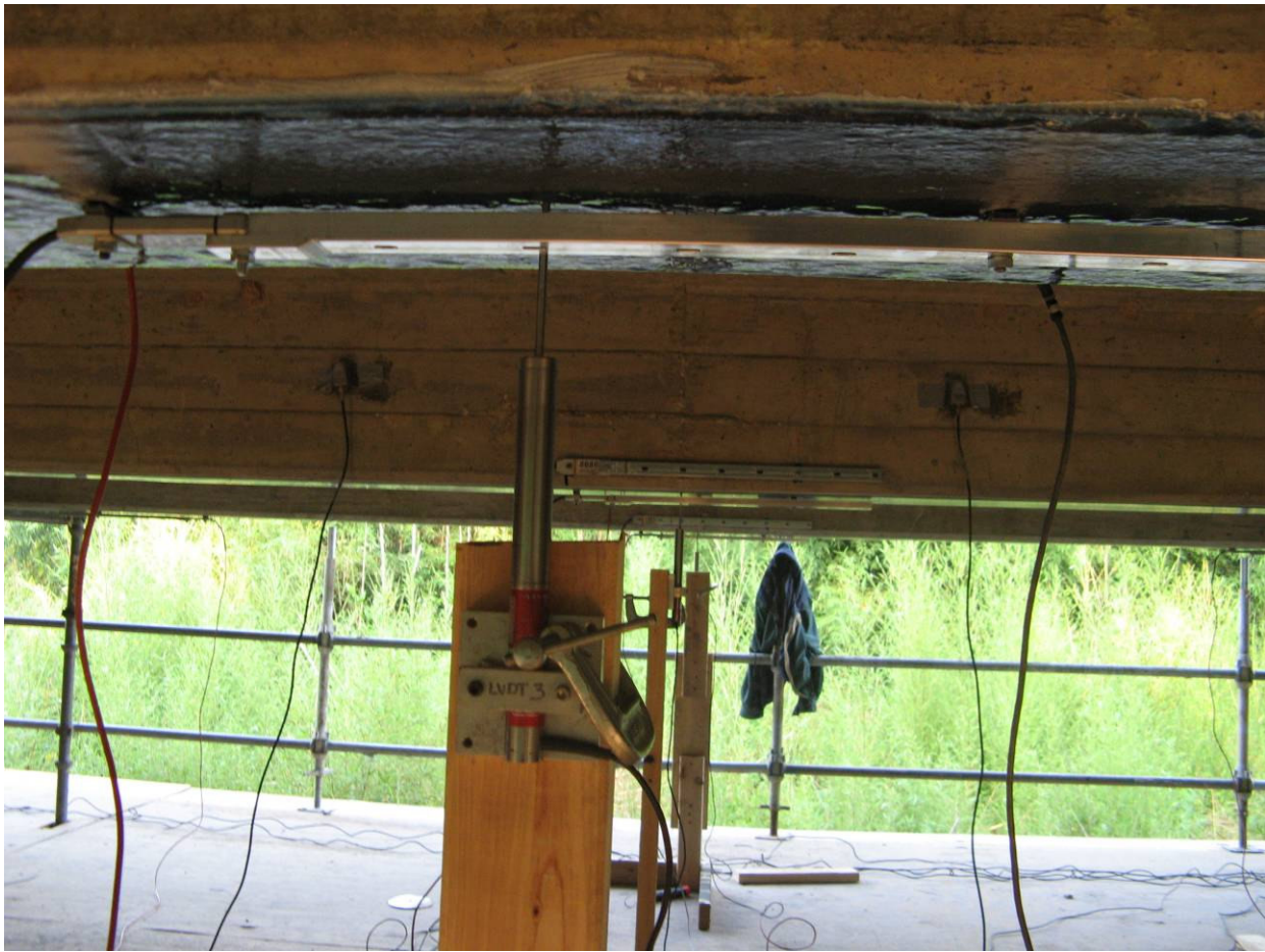
Figure 11 Photograph showing strain and displacement instrumentation.
