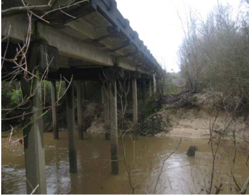
Figure 1 View of sub-structure and super-structure of White Bayou Bridge
