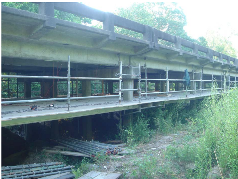
Figure 8 Overall view of White Bayou Bridge
