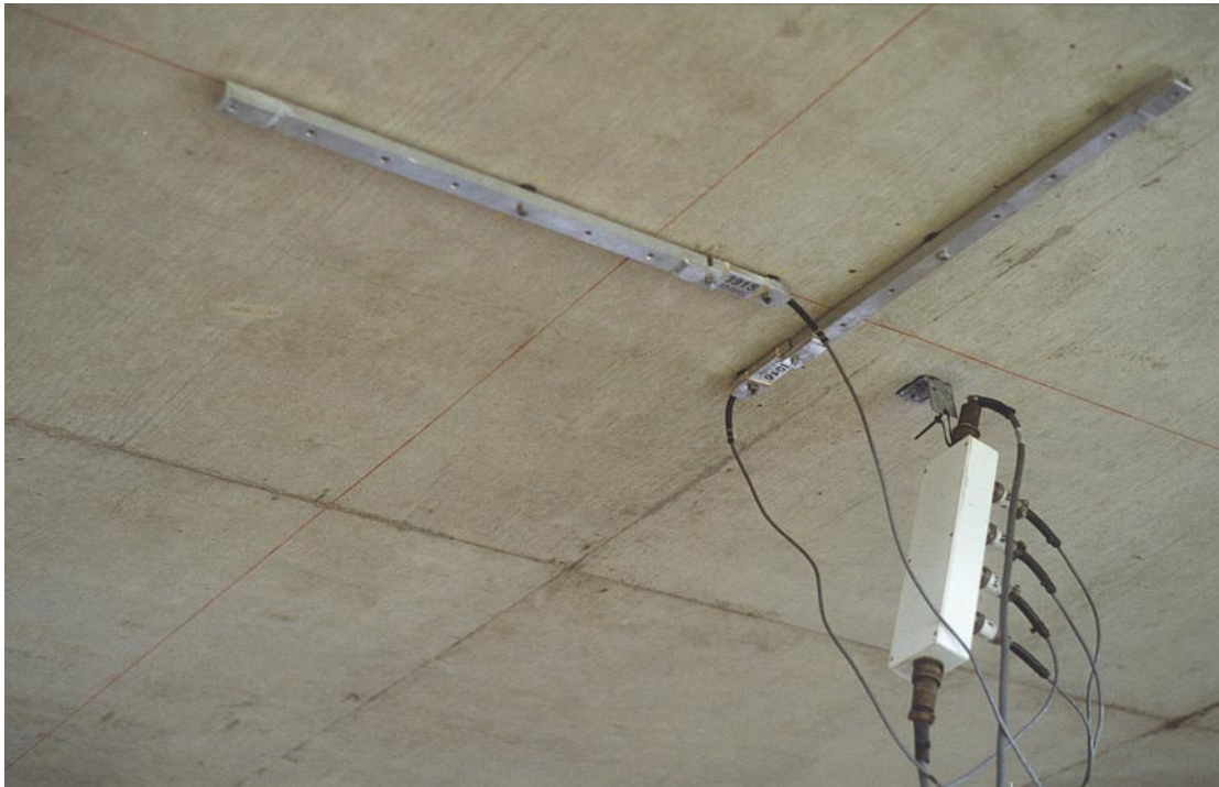
Figure 61 Transducers w/Gage Extensions Mounted On R/C Slab
