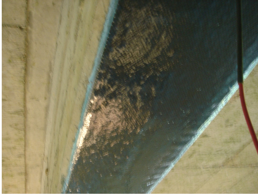
Figure 9 Wet lay-up
