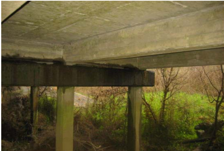
Figure 2 View of pile cap, beam, and deck of White Bayou Bridge
