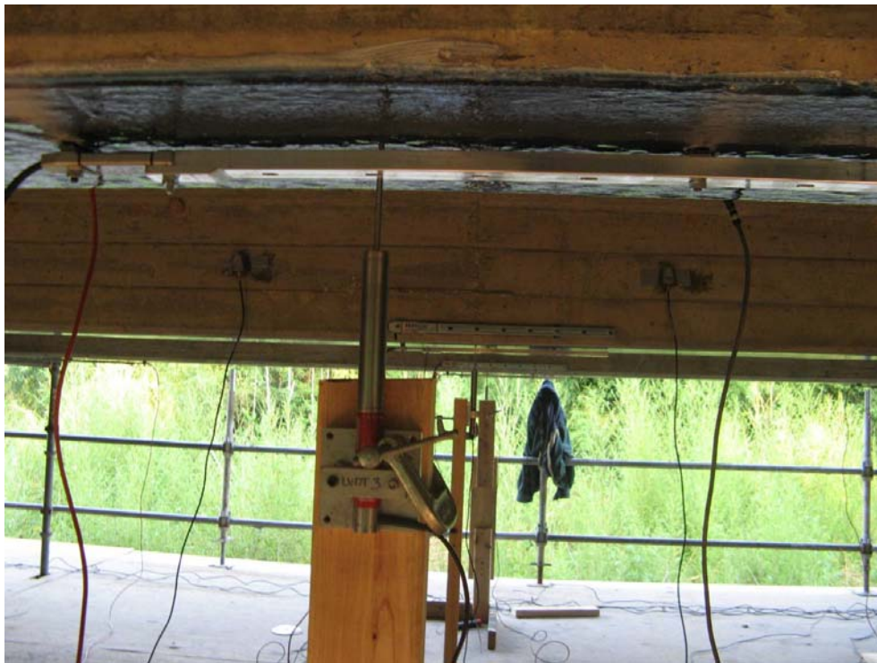
Figure 21 Photograph showing strain and displacement instrumentation
